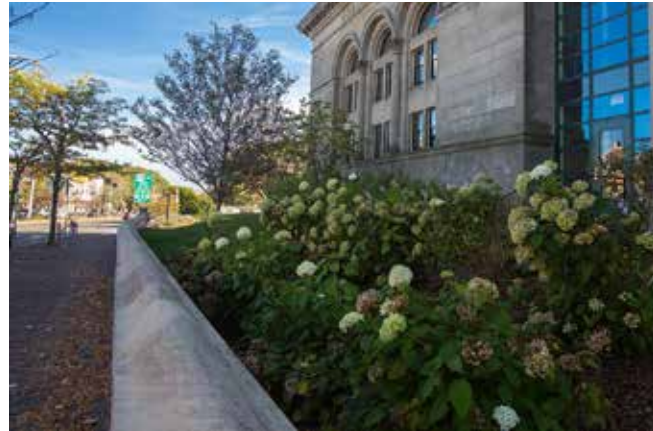
Olmsted Brothers civic block garden wall restoration.
