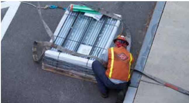
Solar panel installation at Dallin School.
