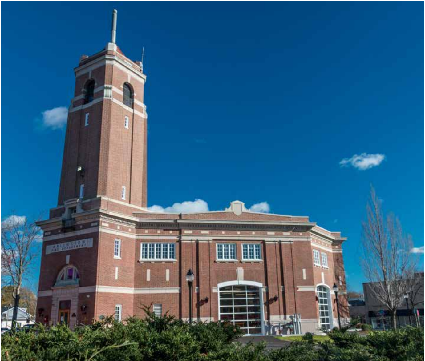
Renovated Central Fire Station and new AFD Headquarters
