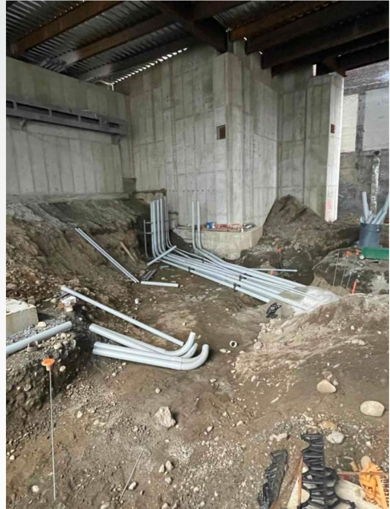
Underground Plumbing & Electrical
