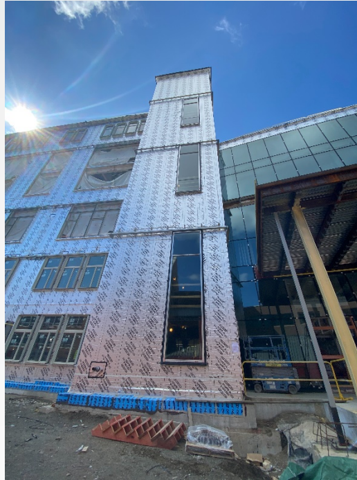
Stair 1 Exterior AVB + Curtainwall Glass (BLDG B; Main Entry)
