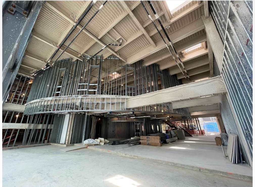
5 th Floor Radius Wall Bldg. B
