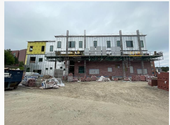
BLDG C – Exterior East Elevation
