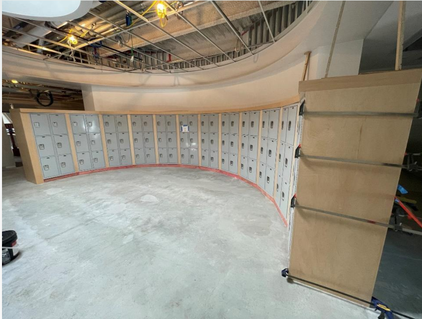
Locker Pod Millwork (BLDG B)
