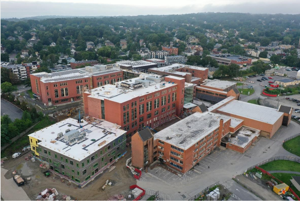
BLDG B + C – Drone
