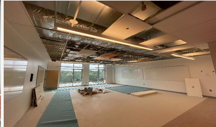
BLDG B Classroom Finishes + Lighting
