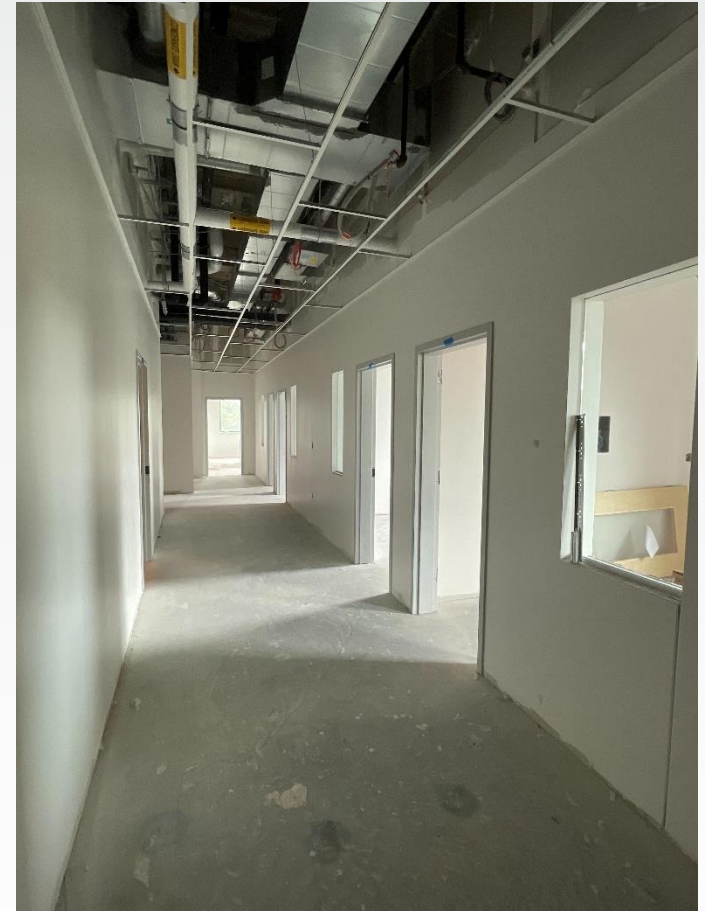
BLDG C Level 2 Boarding + Finishes
