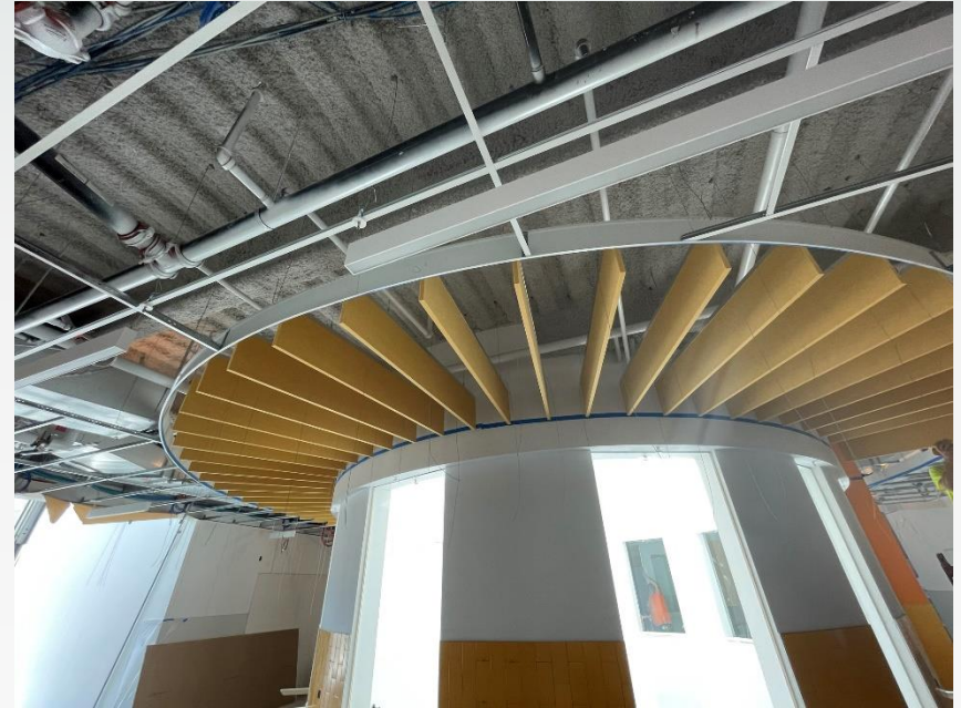
Corridor Ceiling Baffles (BLDG B – Elliptical Lightwell)
