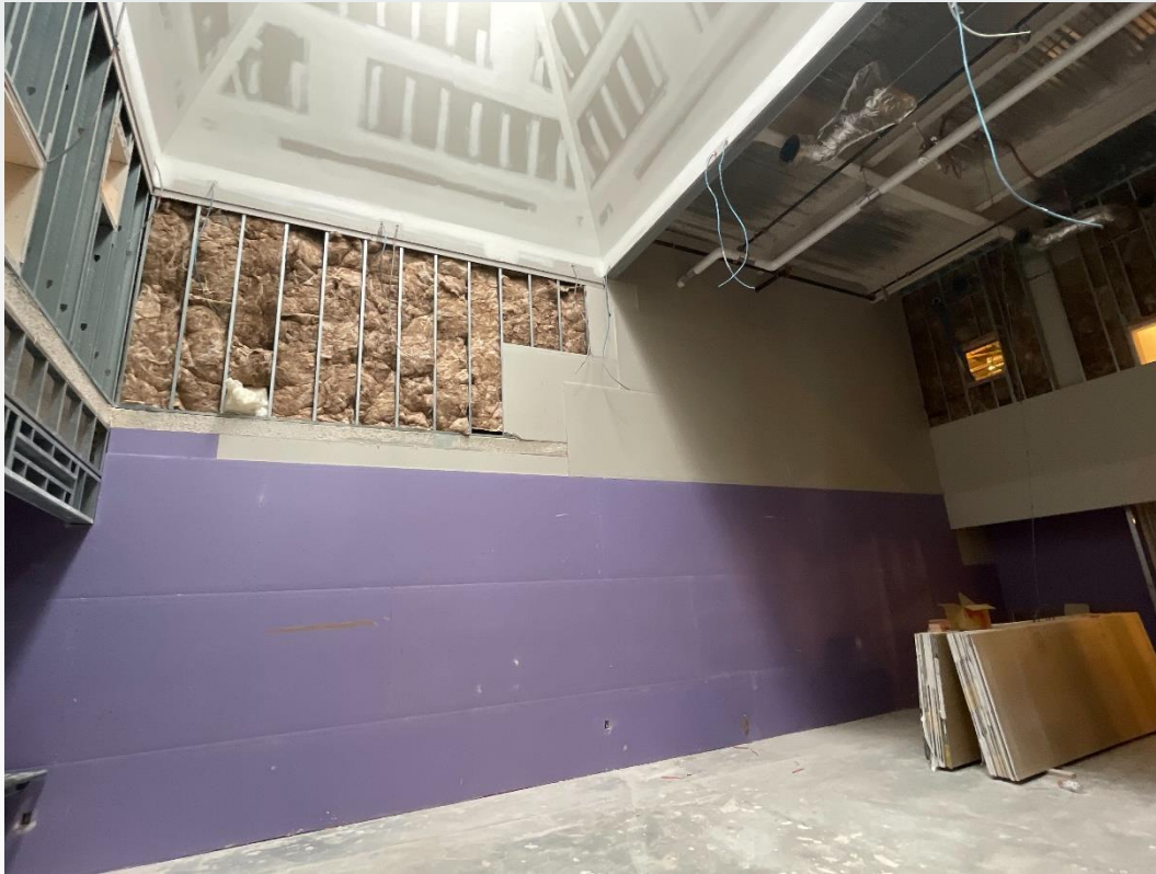
BLDG C – Levels 1 + 1.5 Framing + Progress (Multipurpose Room)
