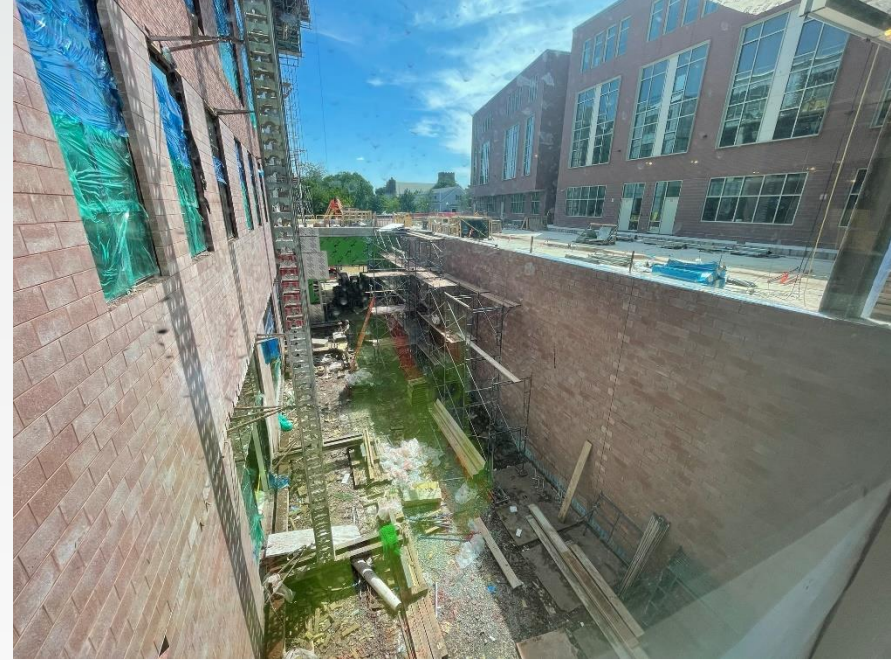
BLDG B Interior Courtyard
