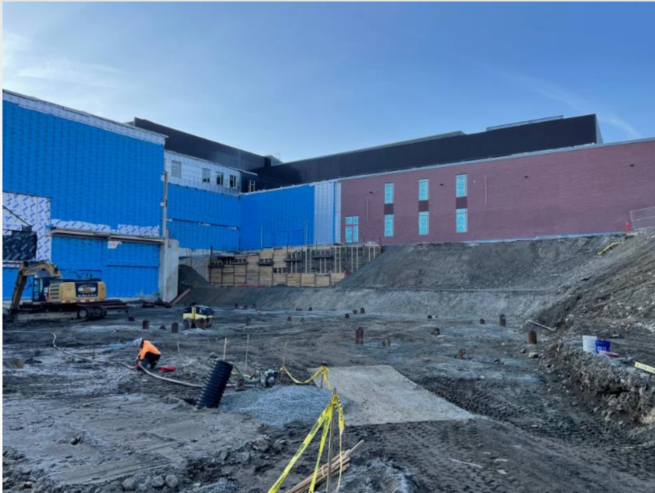
PIF Installation Ongoing (PH 3)
