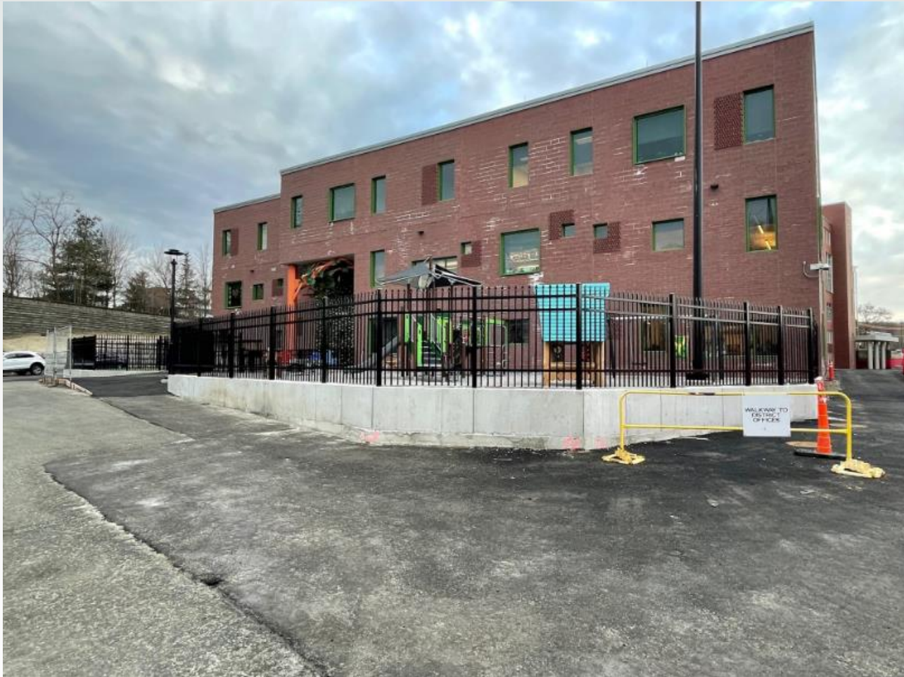
Permanent Fencing Installed at Pre-K (PH 2)
