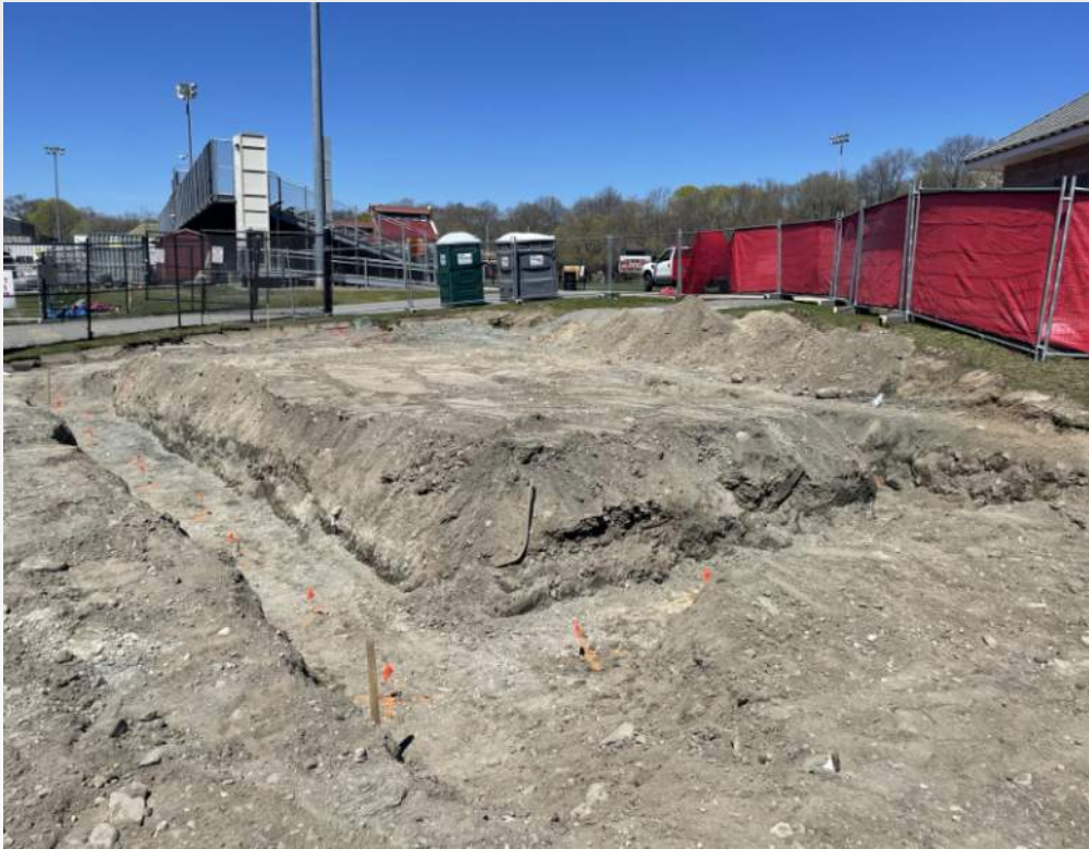
Toilet Building Pre-Ex + Helical Piles
