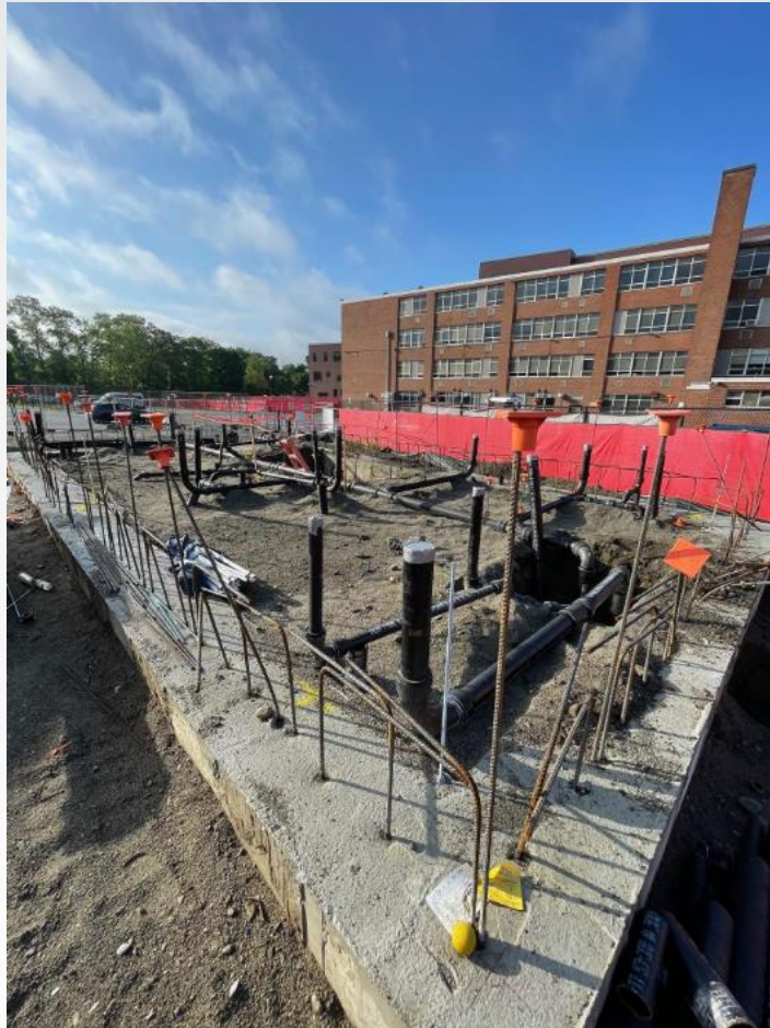
Toilet Building Progress (Foundations + Underground MEP's) (PH 4)
