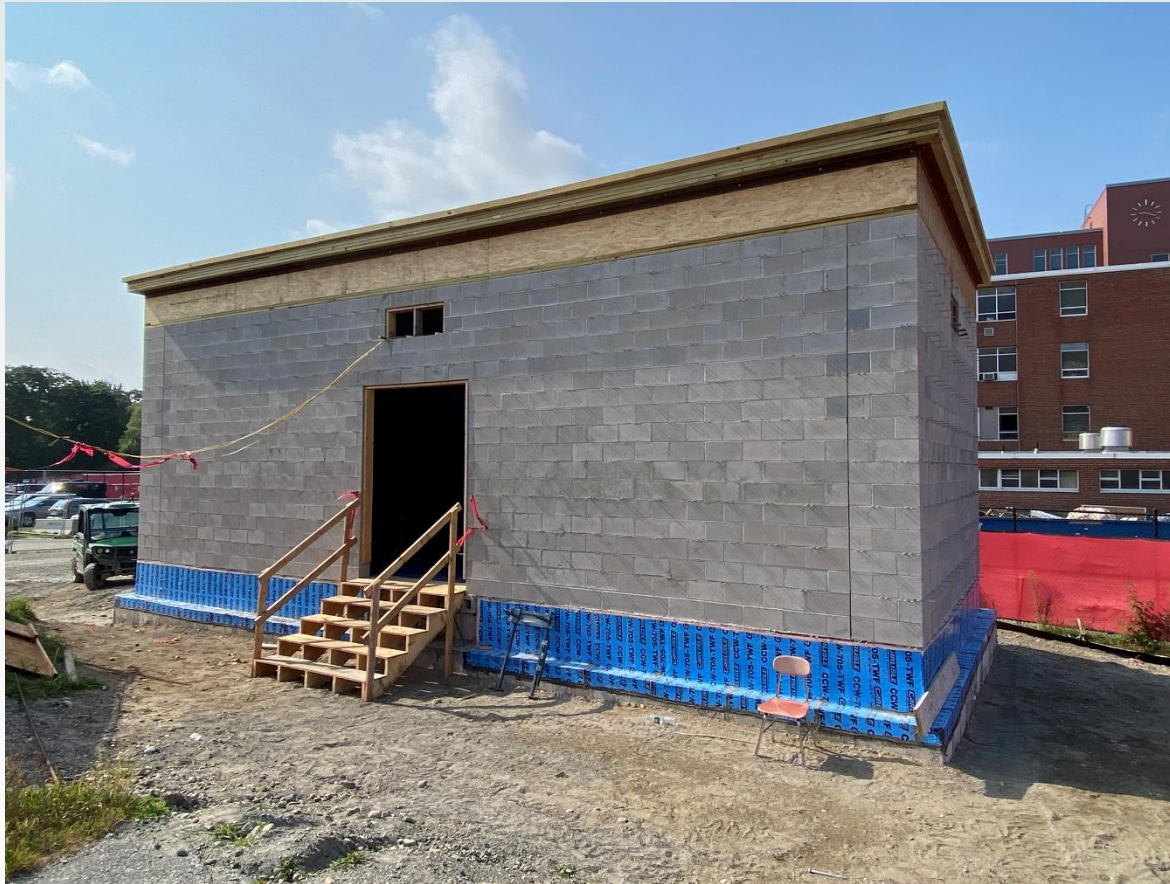
Toilet Building Progress (Masonry) (PH 4)
