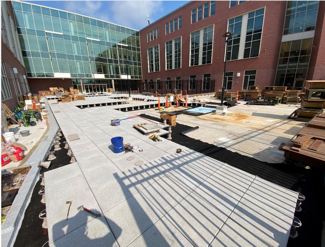
Upper Courtyard Roof Work Ongoing (PH 2)
