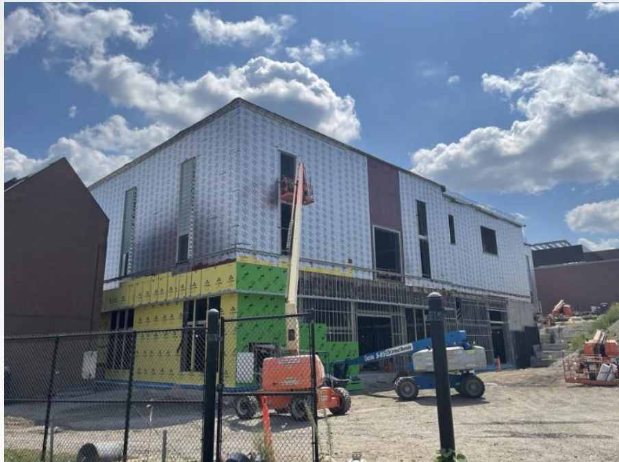
Exterior Framing/Sheathing/CW Install (PH 3)
