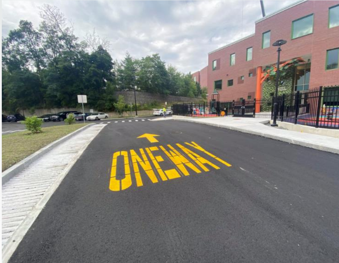
PreK East Parking Lot Final Pavement (PH 2)
