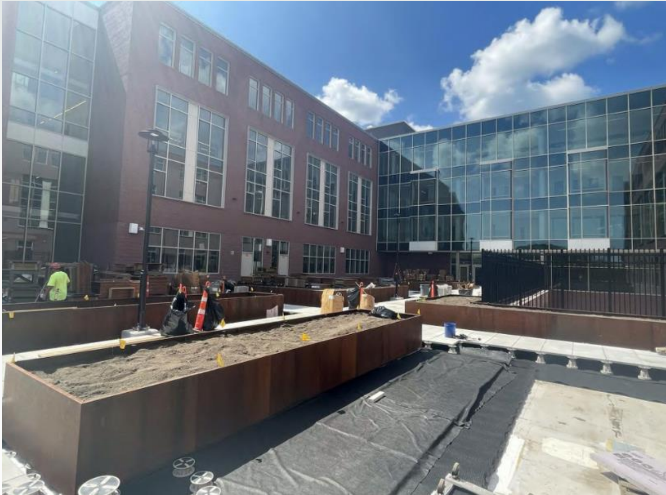
Upper Courtyard Roof Work Ongoing (PH 2)
