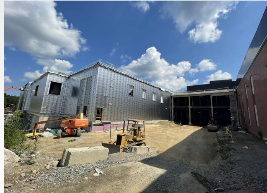
Exterior Framing/Sheathing/CW Install (PH 3)
