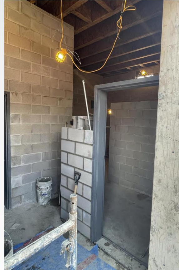
Toilet Building Progress (MEPs + Interior Masonry) (PH 4)
