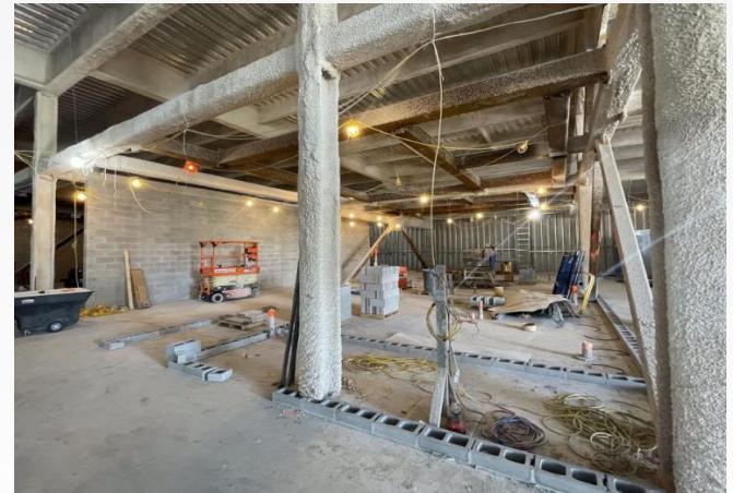
Level 1 + 2 Interior Framing + Masonry Partitions (PH 3)
