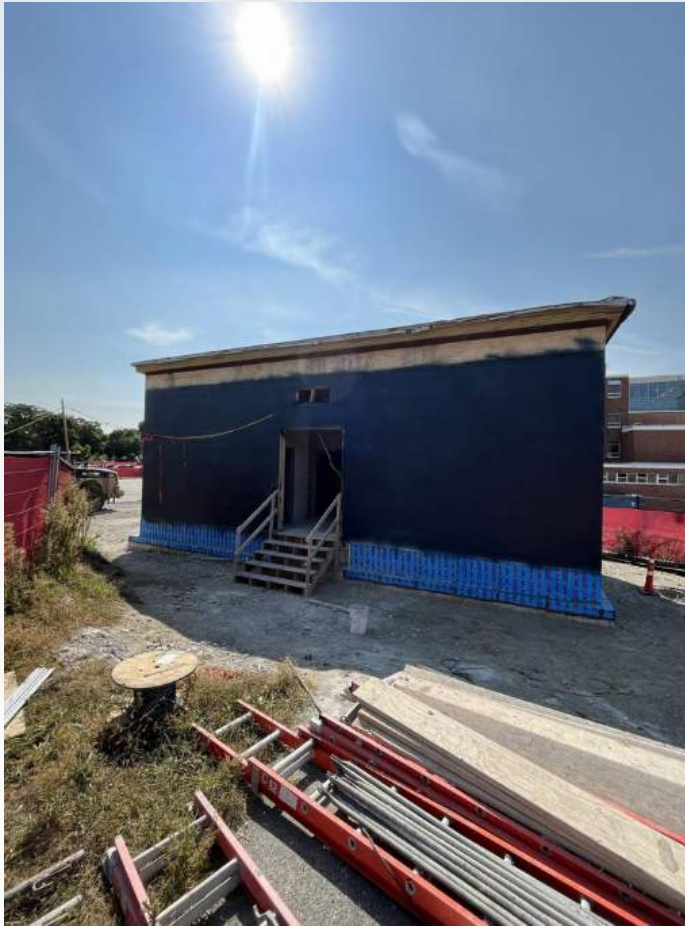
Toilet Building Progress (Waterproofing + Interior Masonry) (PH 4)
