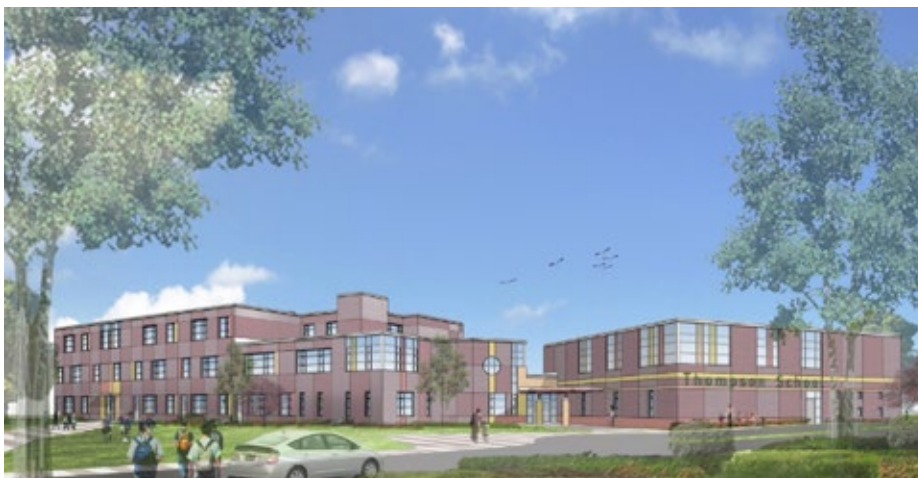
North entry view of upcoming Thompson Elementary School
