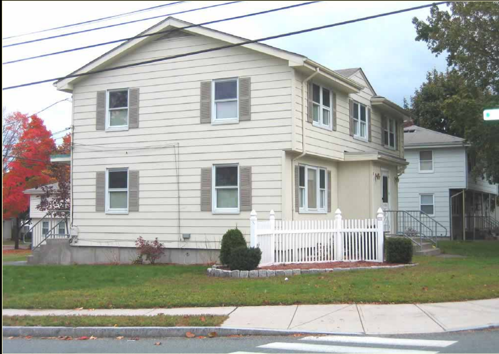
Building that is too close to the street
