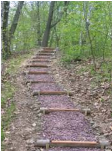
Pathway stabilization at Window on the Mystic, 2005
