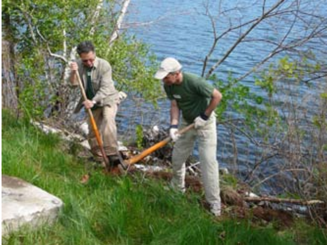
Preparing to dig into Spy Pond hillside for the bench
