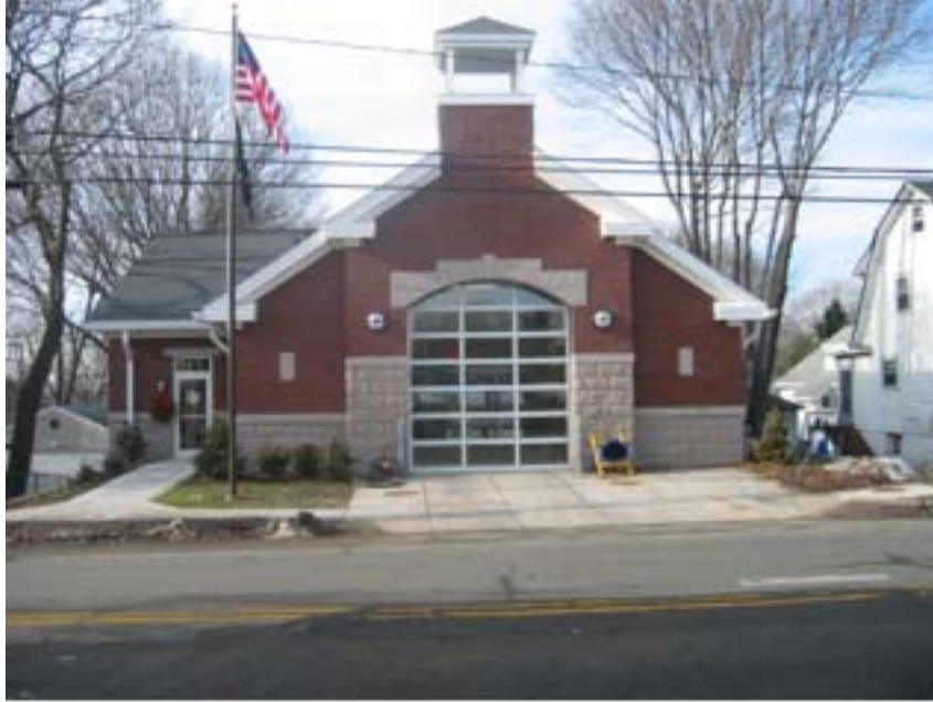
Park Circle Fire Station
