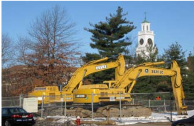
CVS construction site
