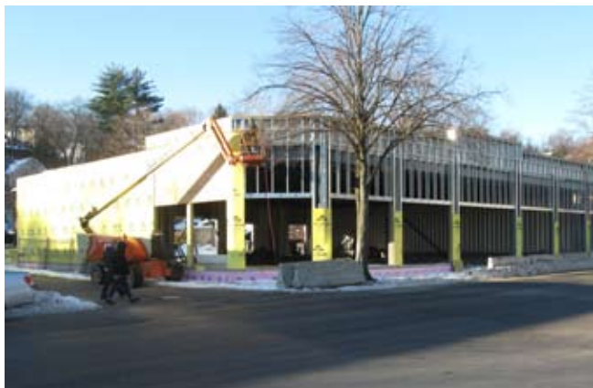
Arlington Heights Retail Construction
