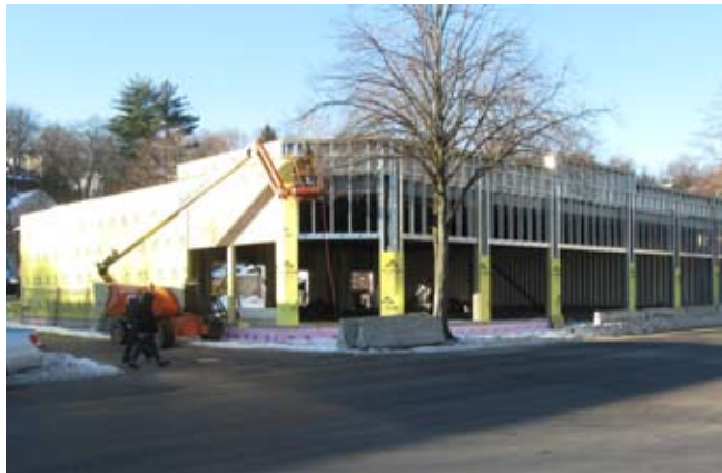
Arlington Heights Retail Construction
