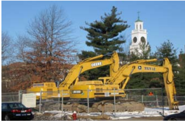
CVS construction site
