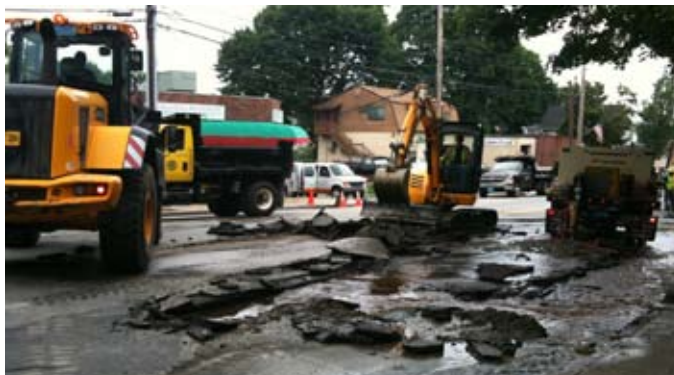
Repair operations on water main break in Arlington Heights
