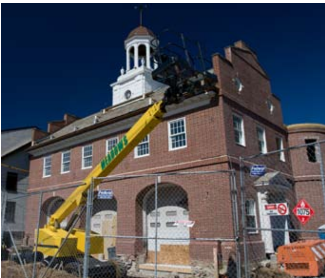
Highland Station construction
