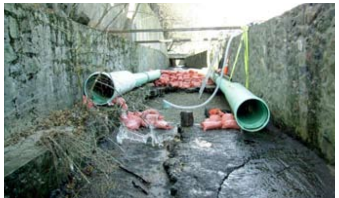
Emergency repair site of Mill Brook Culvert by Ryder Street.
