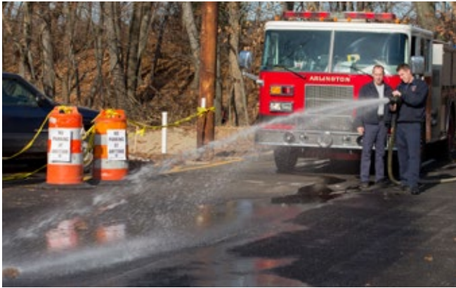
AFD demonstrate porous pavement at Hurd Field parking lot.
