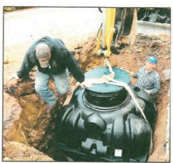
COURTESY PHOTO A large storage tank was recently installed at the Rockport Community House to harvest rainwater for use in irrigation.
