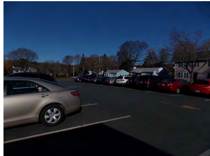
The parking lot has also been repaved and is in good condition.
