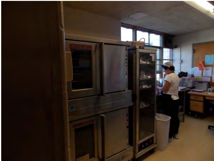
The food preparation area is undersized; it is currently located in a renovated office.
