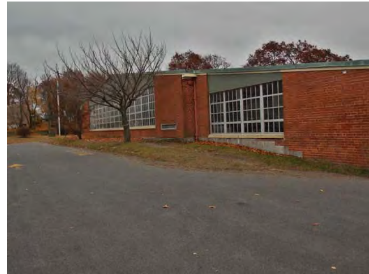
Three kindergarten classes are also located in the original building. Note the large windows are all metal framed single glazed.
