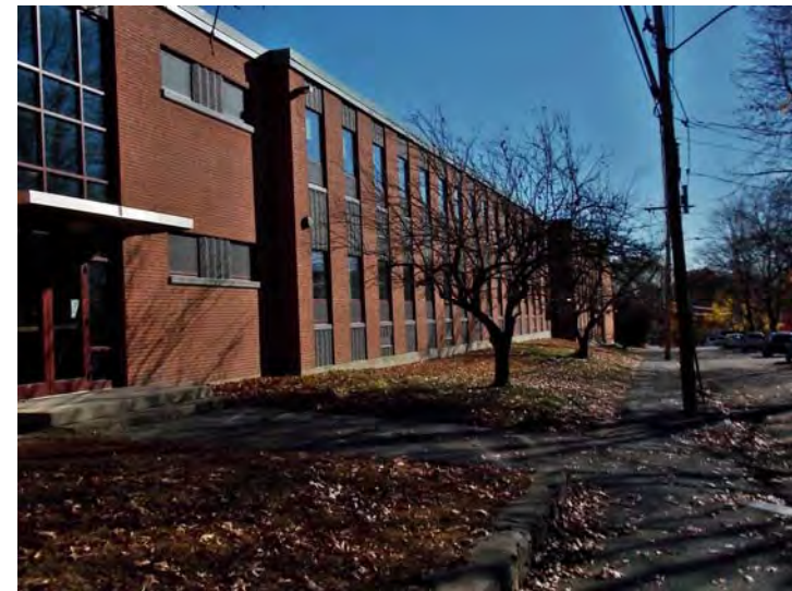
The new (renovated) wing has two levels, brick exterior walls and metal-framed double glazed insulated windows.
