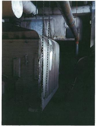
5. Existing ACM insulation on Boiler #2, associated piping and ductwork to be removed will be abated by Owner. Contractor shall abate ACM within boiler sections and other ACM incidental to the work of this contract.
