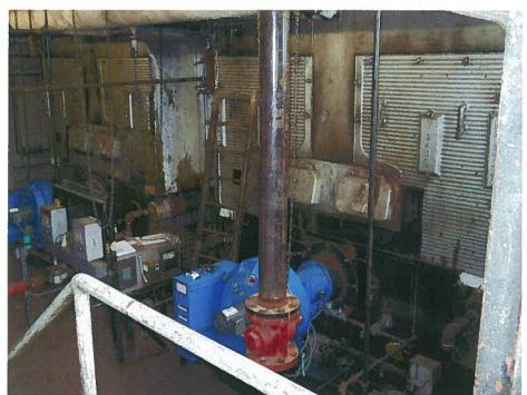
Overall view of F Boiler Room from stair landing. Replace existing boiler and accessories on the right with new. Protect existing boiler and accessories on the left from damage caused by the work of this contract.
