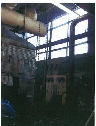
4. Existing window adjacent to the existing Boiler #2 to be removed. At Contractor's option, this window maybe temporarily removed, salvaged, stored and reinstalled, if necessary, for removing the demolished boiler from the Boiler Room.
