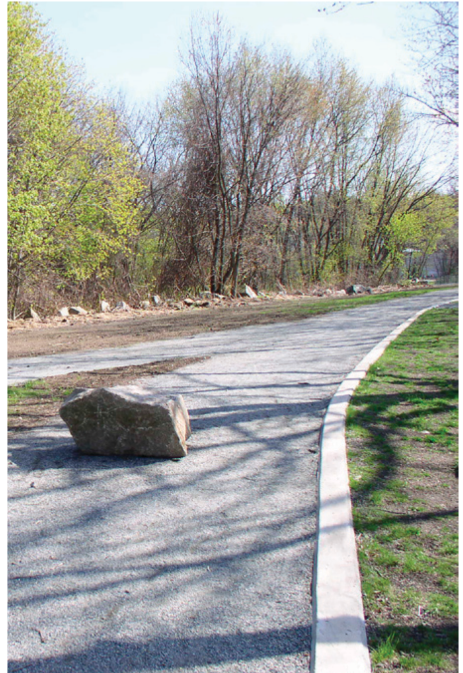
Upgrades to Arlington Reservoir
