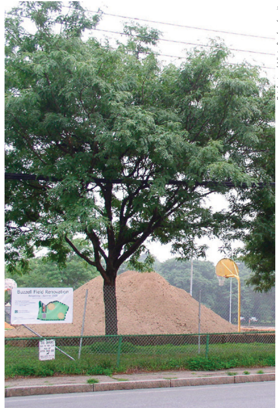
Buzzell Field undergoing renovations
