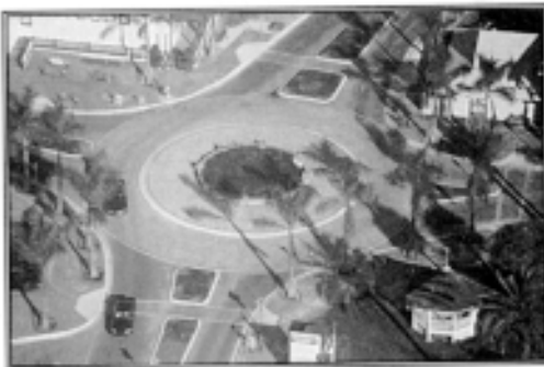
This Fort Pierce, Florida, roundabout was constructed to reduce speeding, improve safety, and enhance the aesthetics of the community.
