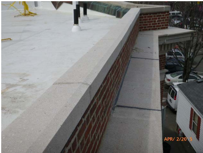
Photo of repaired vertical joint and horizontal joint.
