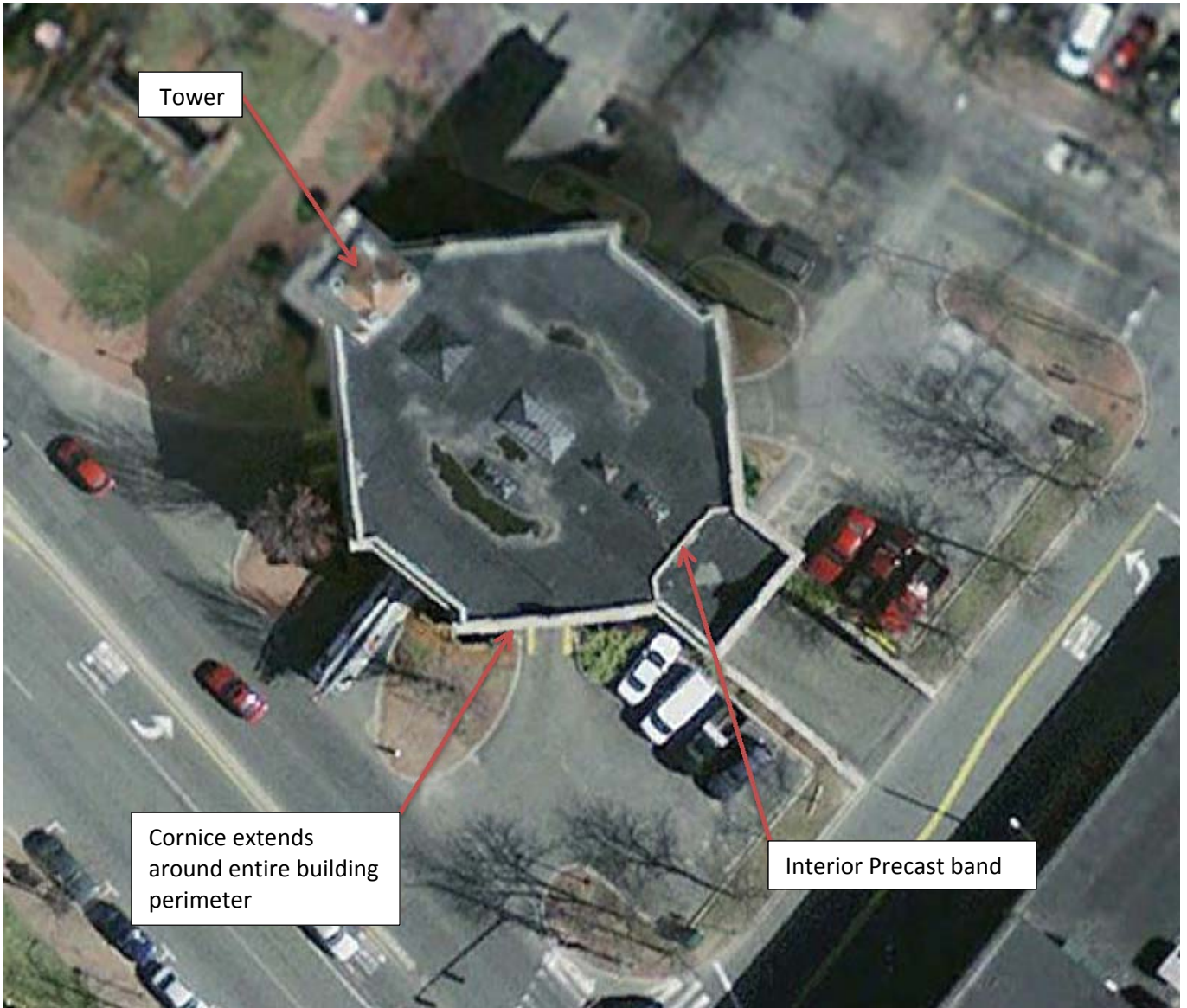
Aerial photograph showing the Central Station in context with repair work.
