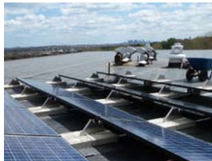
Solar Panel Installation at Ottoson.
