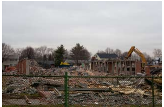
Thompson School Demolition
