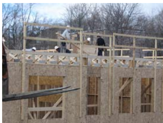
Construction of apartments at 30-50 Mill Street
