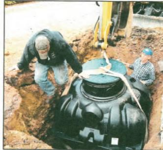
A large storage tank was recently installed at the Rockport Community House to harvest rainwater for use in irrigation.
