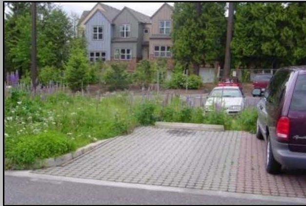
Porous Paver Parking Stalls
