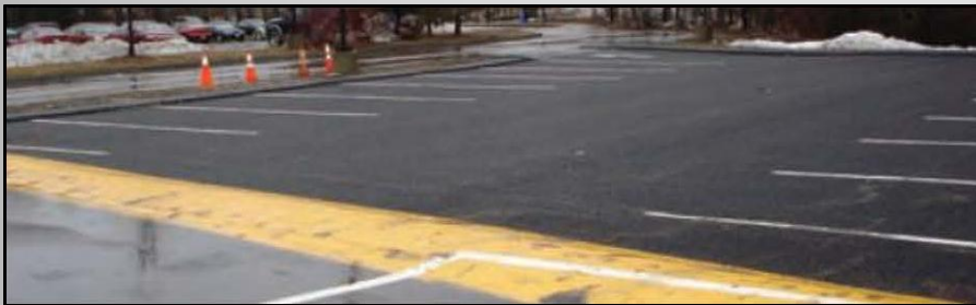
↑ ← Porous Asphalt Parking Lot at UNH, with cross section
