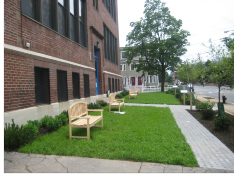
Site after project implementation
