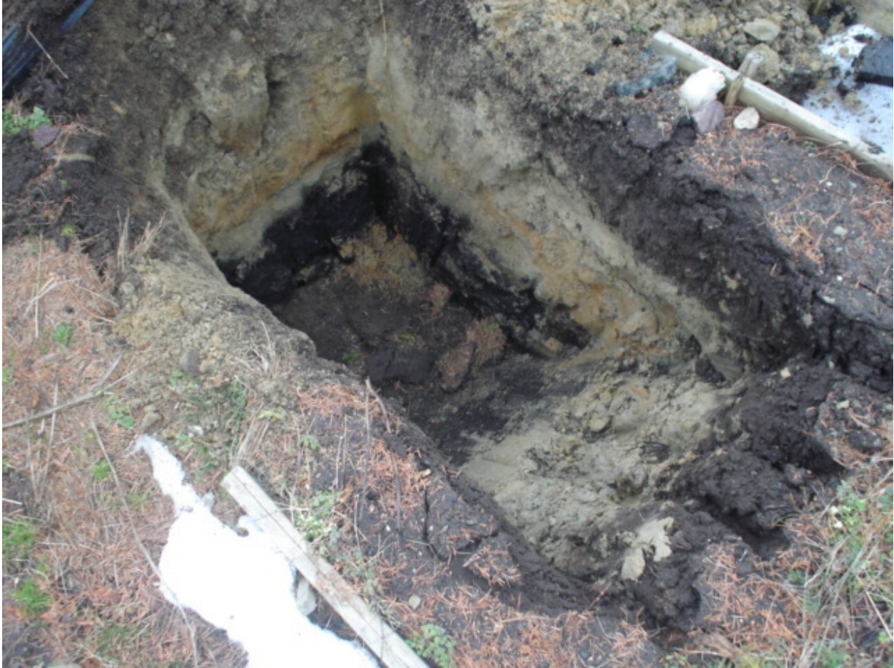
Photo 3 Test Pit TP-3
