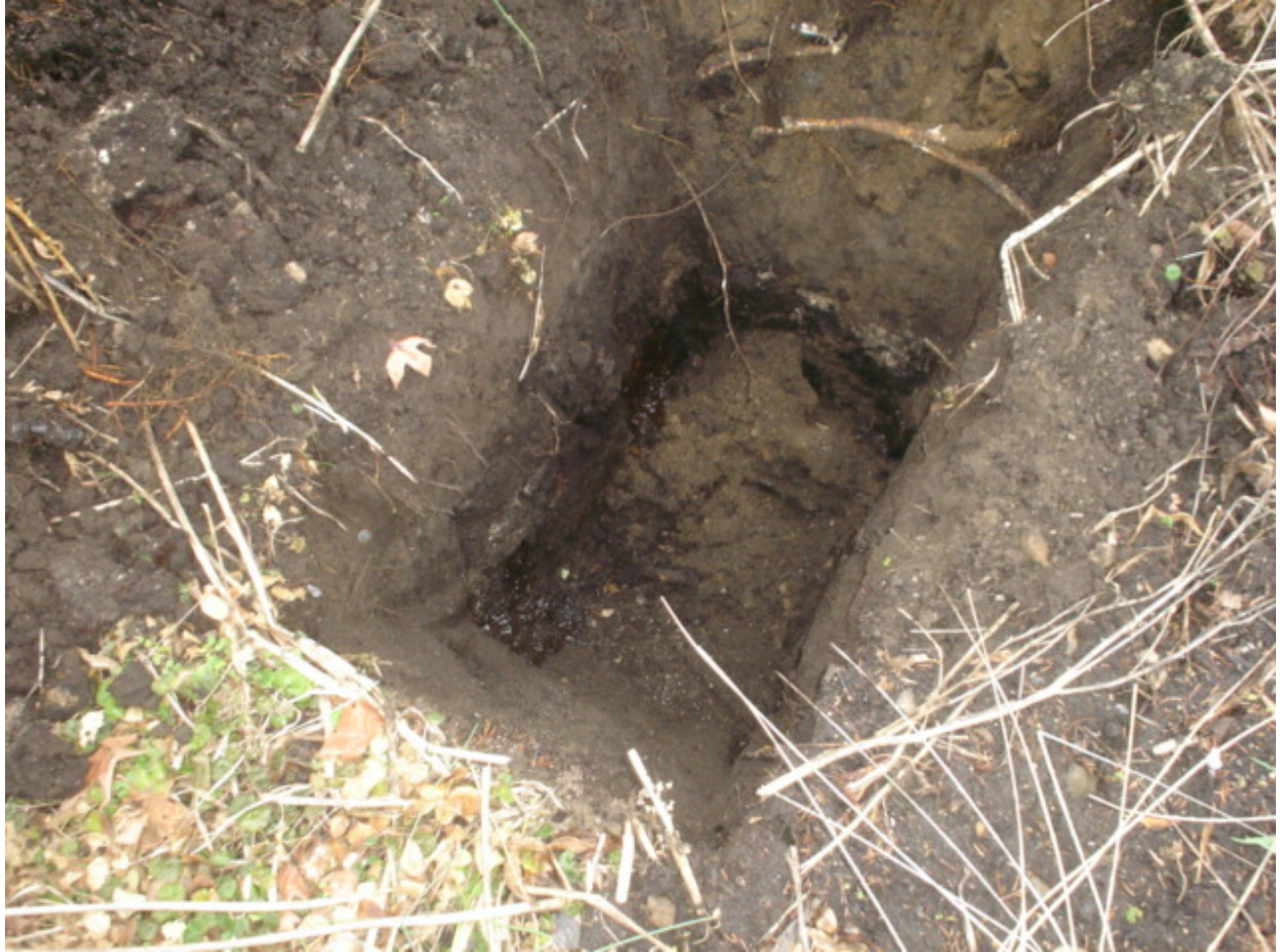
Photo 4 Test Pit TP-4
