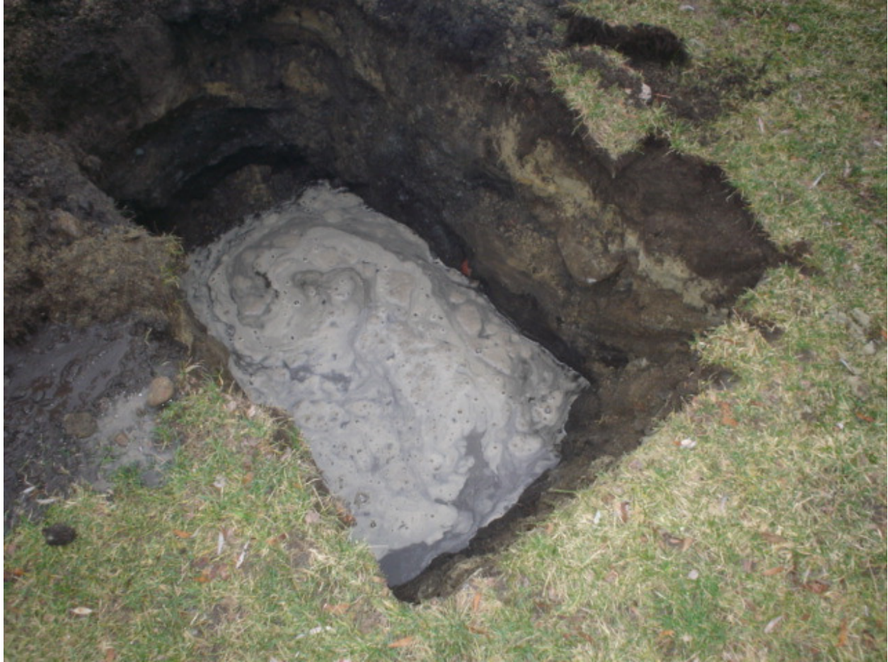
Photo 1 Test Pit TP-1
