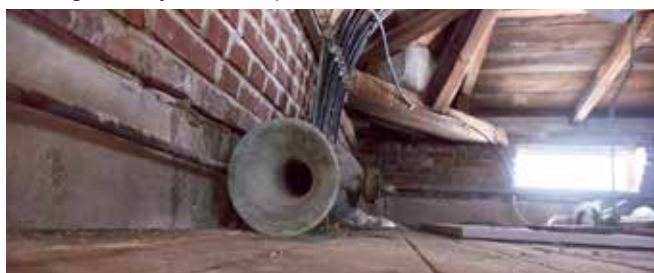
Old firehorn up in Central Station Tower.
