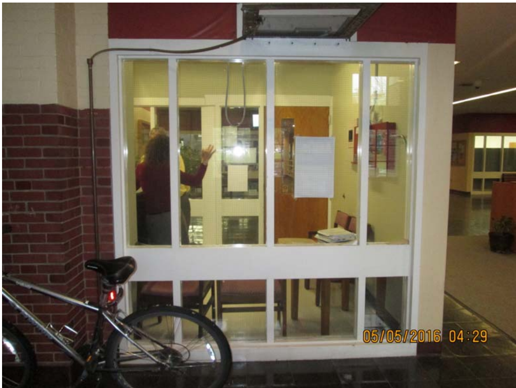
3. Existing Administration Office - viewed from the Entrance Door.
