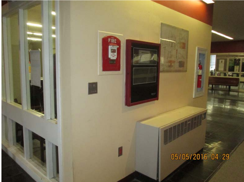
4. Existing Administration Office - viewed from the Entrance Lobby.
