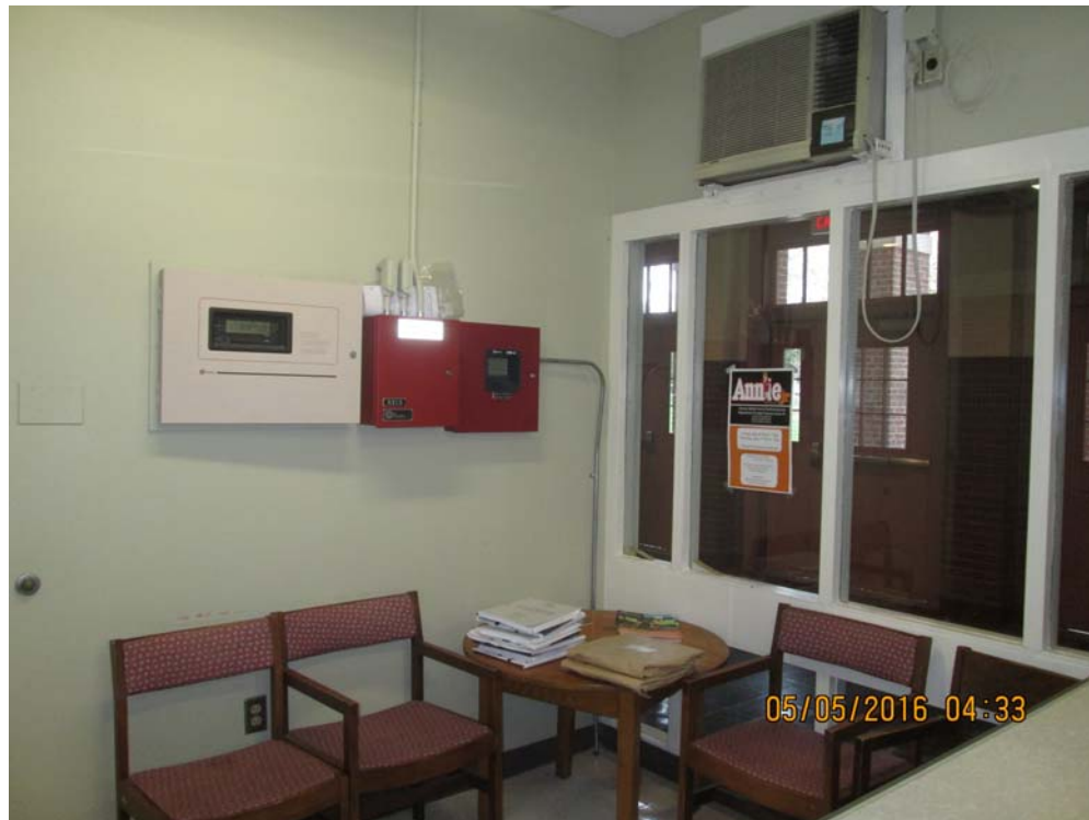
5. Existing Waiting Area at the Administration Office.
