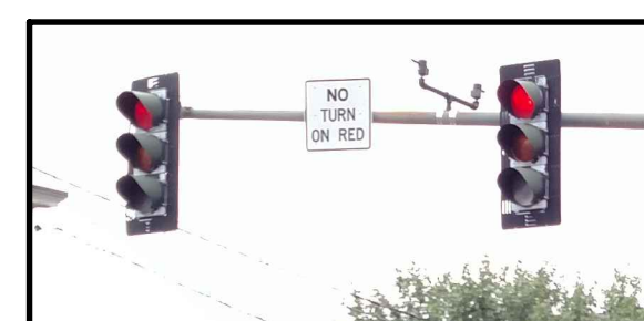
FIG 4b: TYPICAL TRAFFIC SIGNAL HEAD
