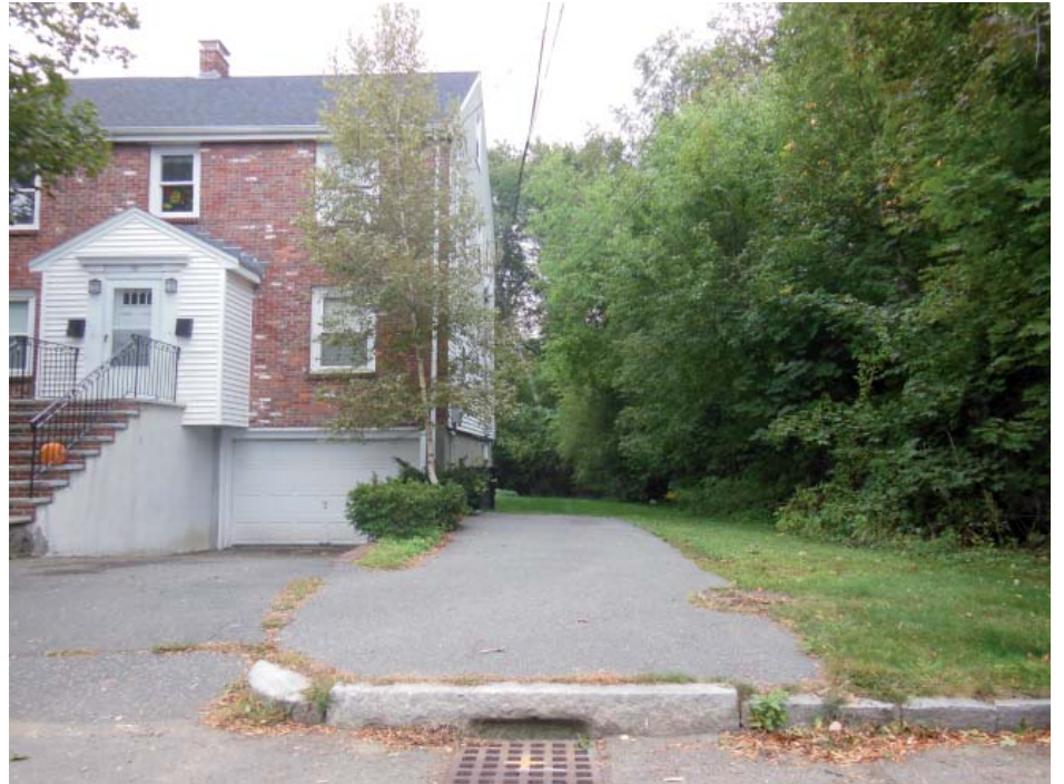
Dorothy Road home adjacent to site.
