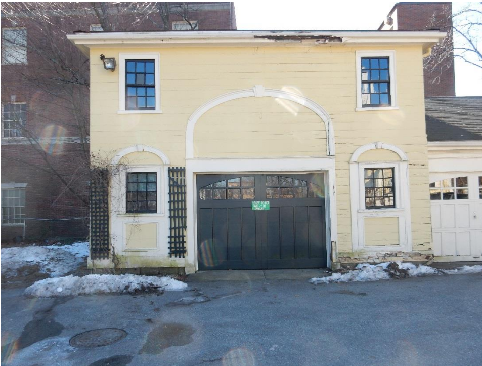
6. North face of two story section. Significant rot is present in gutter, door jamb trim and architrave, skirt trim, and siding around lower right window. Ivy suckers will anchor into siding promoting conditions favorable for rot.
