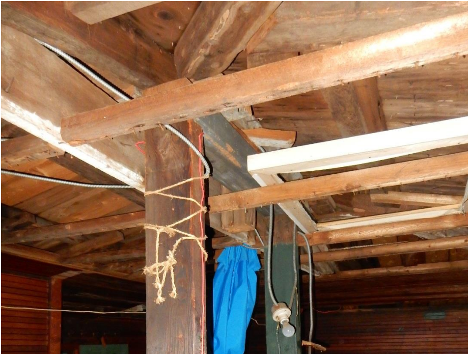
22. Two wood shoring posts support the ends of a 5x5 ridge beam. Ridge beam has a 2x10 lapped and nailed to the sloping 5x5 rafters that align with the ridge beam. This formed a makeshift truss and was the main support for the roof.
