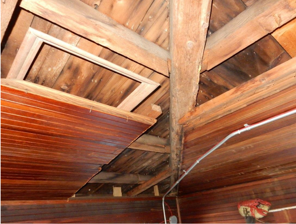
21. Underside of two-story building roof. 3x4 purlins are supported on 5x5 hip beams. Ceiling and walls originally covered with bead board.
