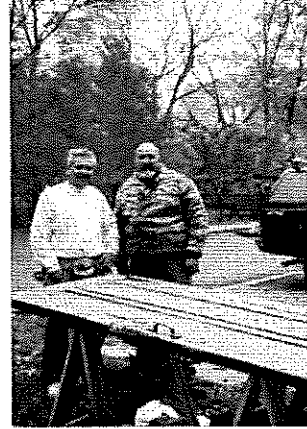
Barn Door being repaired and painted, fall 2014
