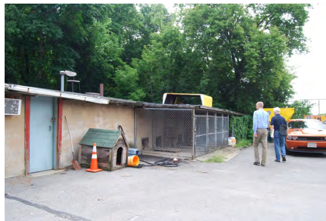
Animal Control Facility impedes DPW functions.
