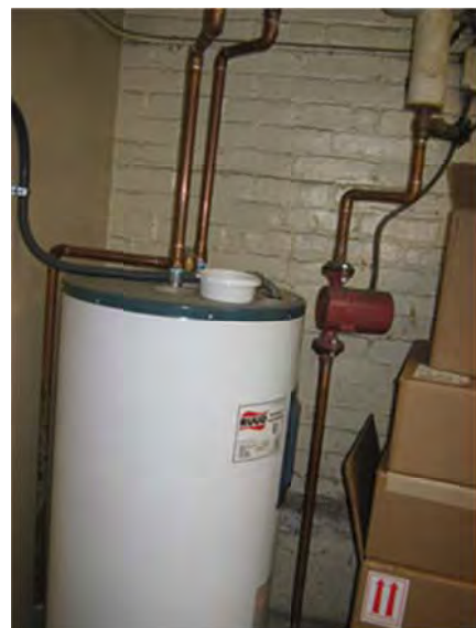
Numerous electric water heaters provide water to hand sinks and fixtures throughout the site.
