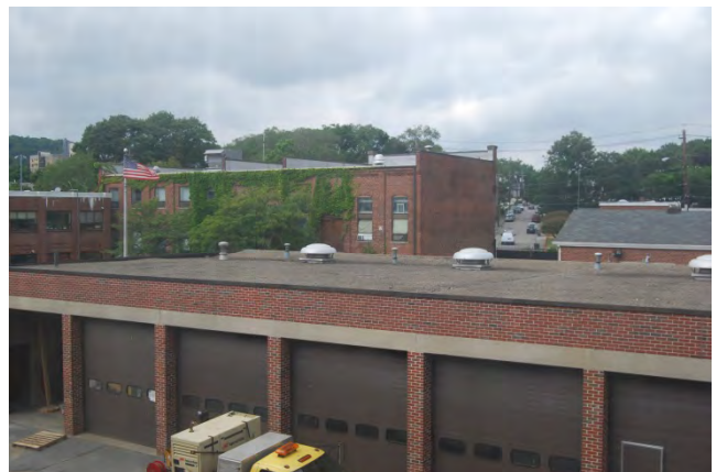
Building C roof after a rainstorm, viewed from Building D roof.
