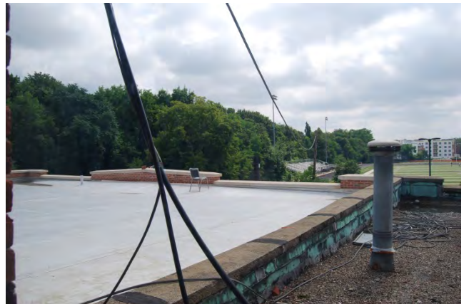
Recently replaced roofing and coping.
