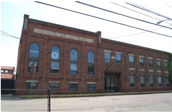
1914 Meter Building (Building A)
