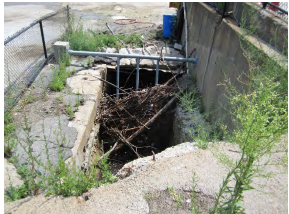
Debris grille in Mill Brook culvert opening.
