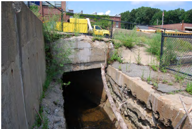
Mill Brook passing through the middle of site.
