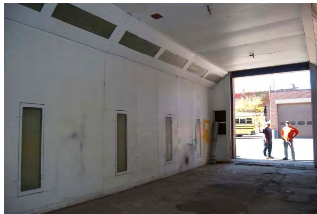
Existing decommissioned paint bay (3) located in Building D
