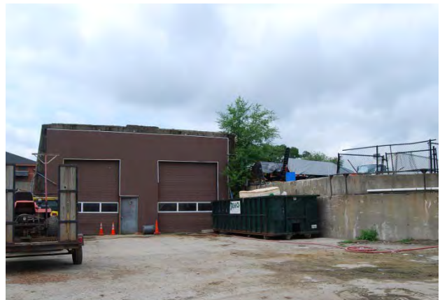
Remaining Transfer Station structure
