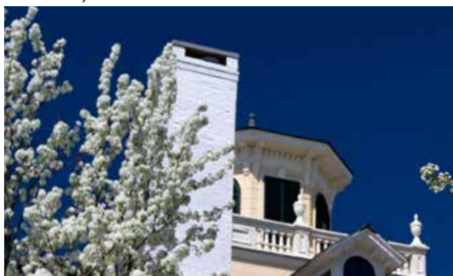
Cupola atop of Whittemore-Robbins House.
