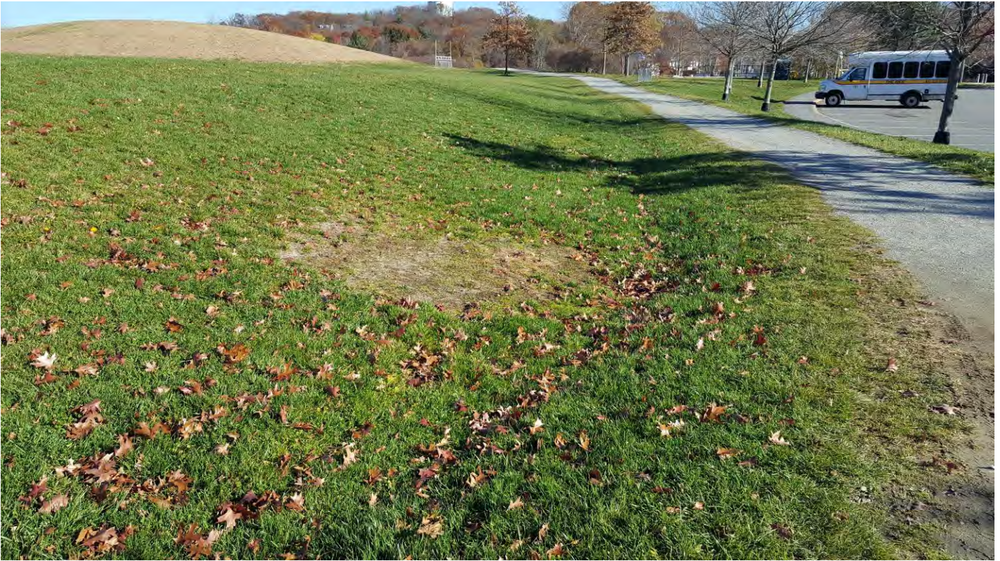
Area of apparent erosion at western portion of property, adjacent to Summer Street parking lot
