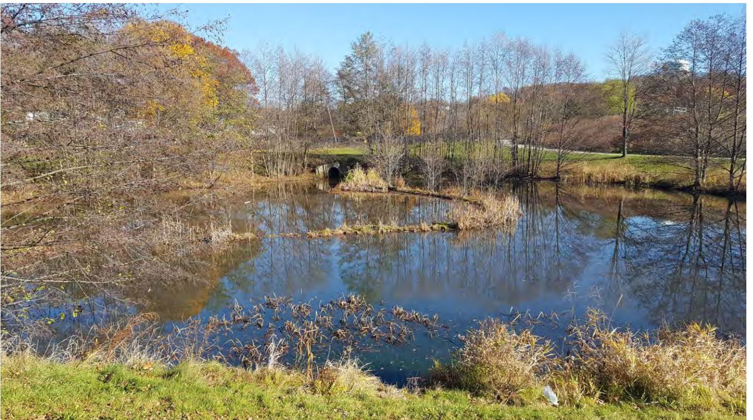
Eastern end of detention basin (facing inlet)
