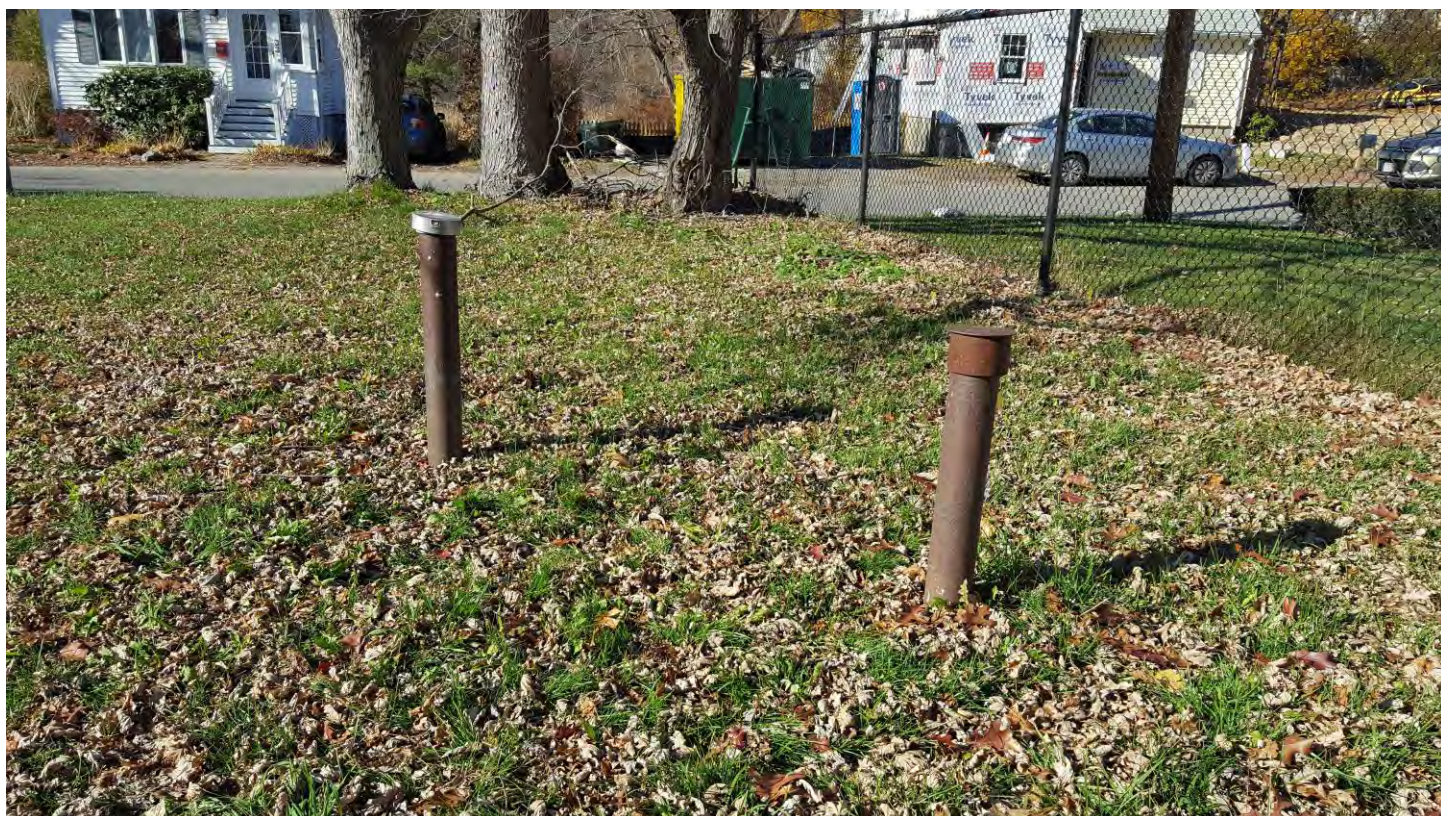
Existing groundwater monitoring wells, adjacent to Reed Street (north side of basin)
