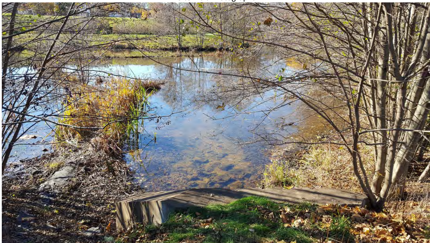
Eastern end of detention basin (facing west, at inlet/headwall)
