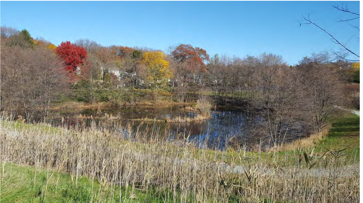
Eastern end of detention basin, facing northeast
