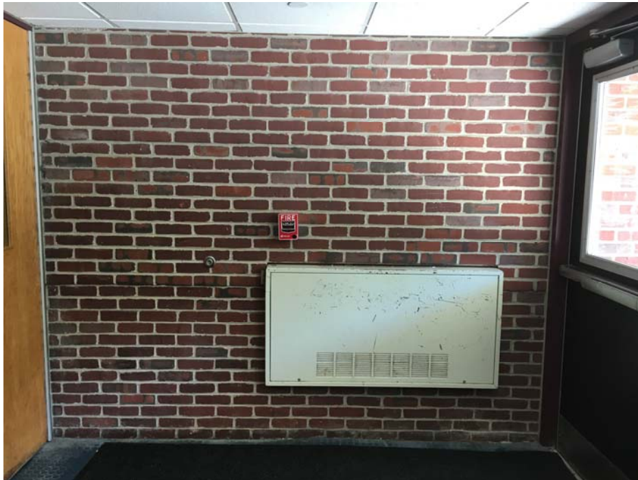
4. Existing entry vestibule wall (opposite side to photo shown above)
