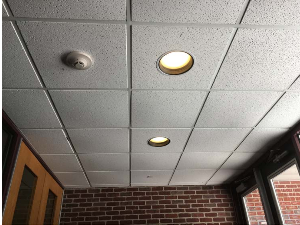
5. Existing vestibule ceiling.
