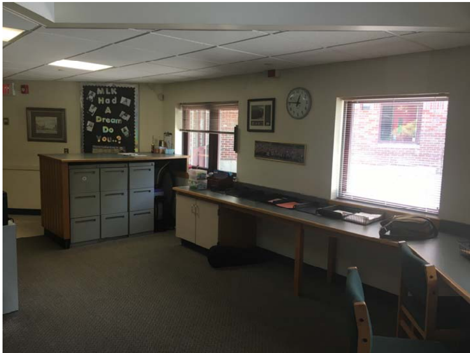
8. Existing Administration Office. Coordinate with owner for removal of existing casework.
