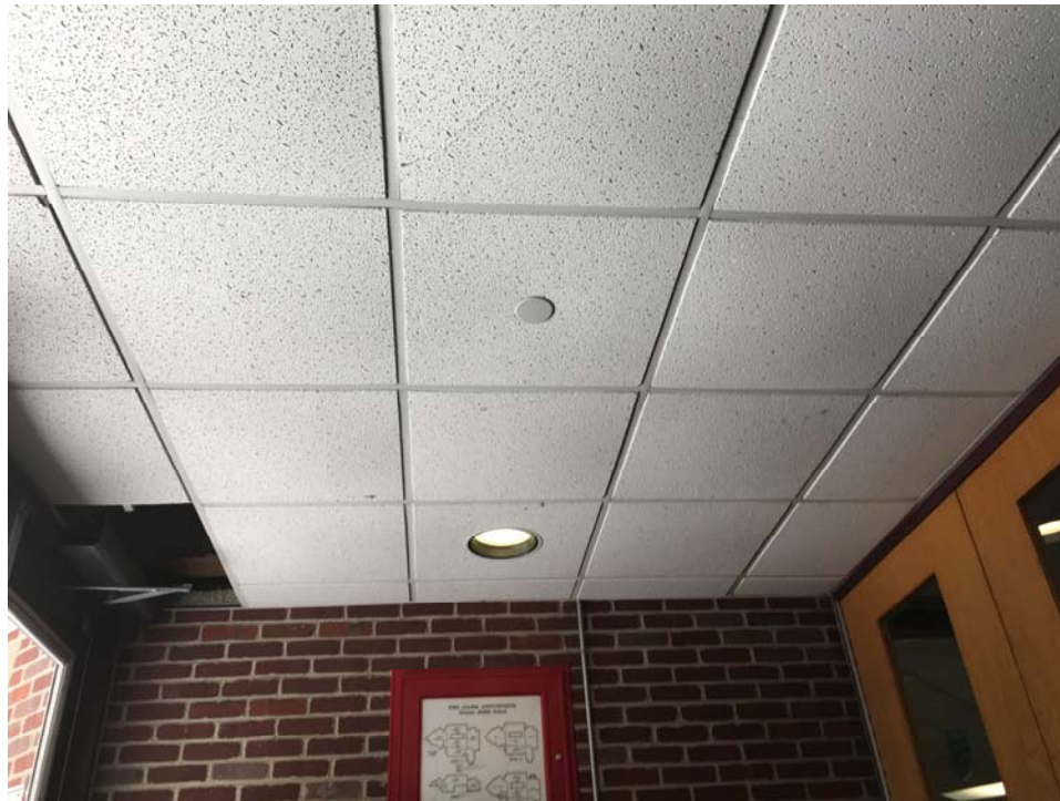
6. Existing vestibule ceiling.
