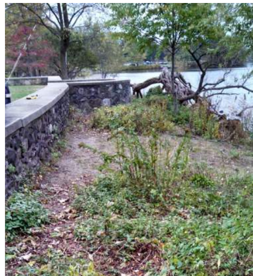
Photograph 8: Foot Path along Stone Wall
