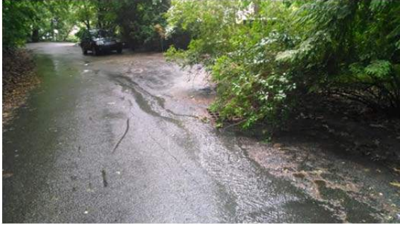
Photograph 14: Uncontrolled Stormwater Runoff
