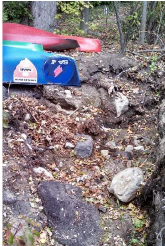
Photograph 17: Eroded Slope at the Uprooted Tree
