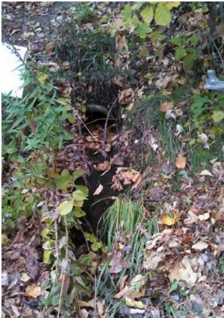
Photograph 13: Obscured 12-inch Stormwater Outfall
