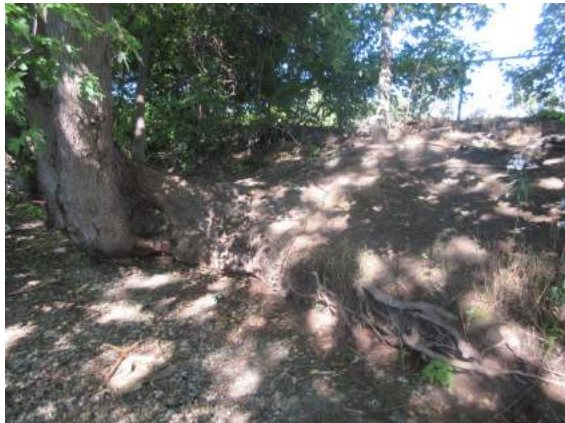
Photograph 2: Erosion with Visible Undercutting
