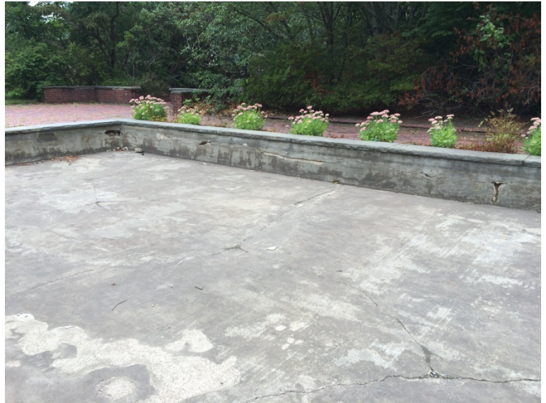
Failing Basin Pool Walls
