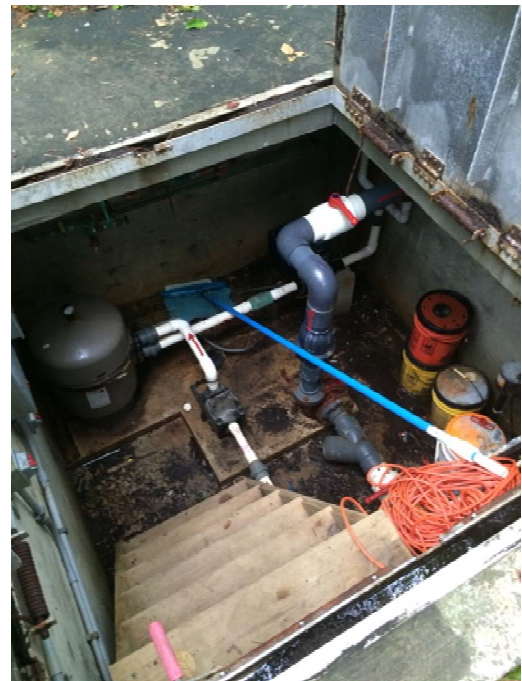
Current Vault Conditions
