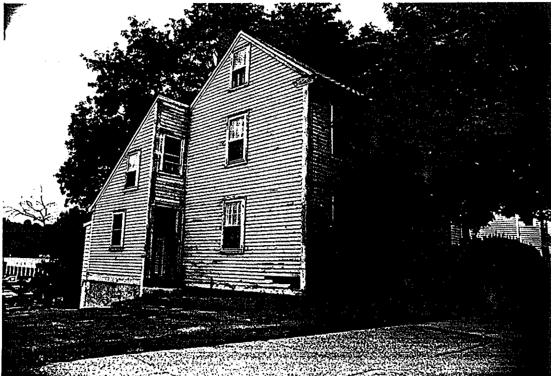
2. West elevation at previous site after aluminum siding had been removed.
