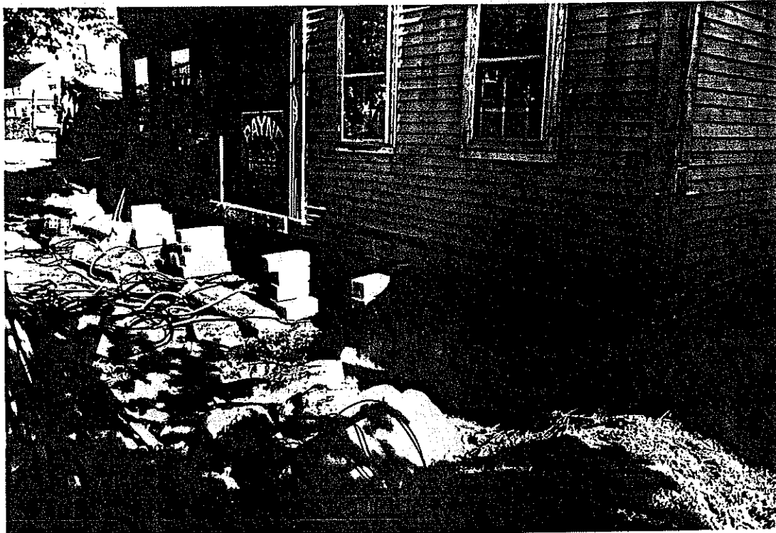
4. Front of house showing cribbing prior to the move.
