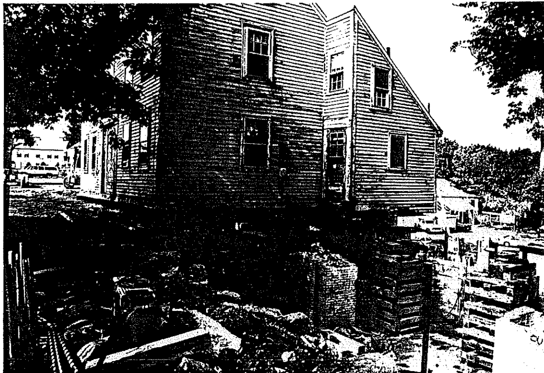
6. The house moved off its previous foundation.
