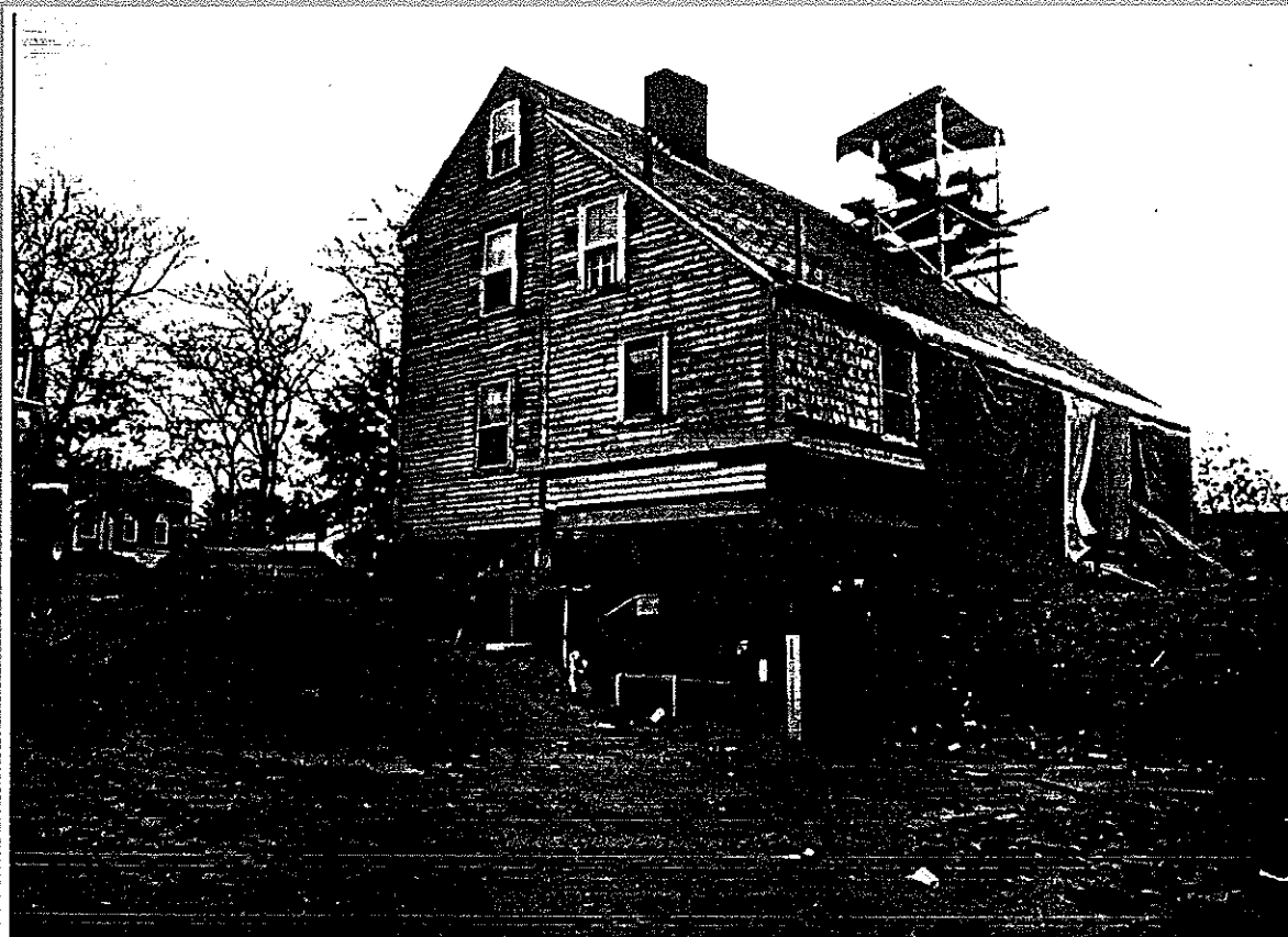
8. Rear of structure showing new sills being installed.
