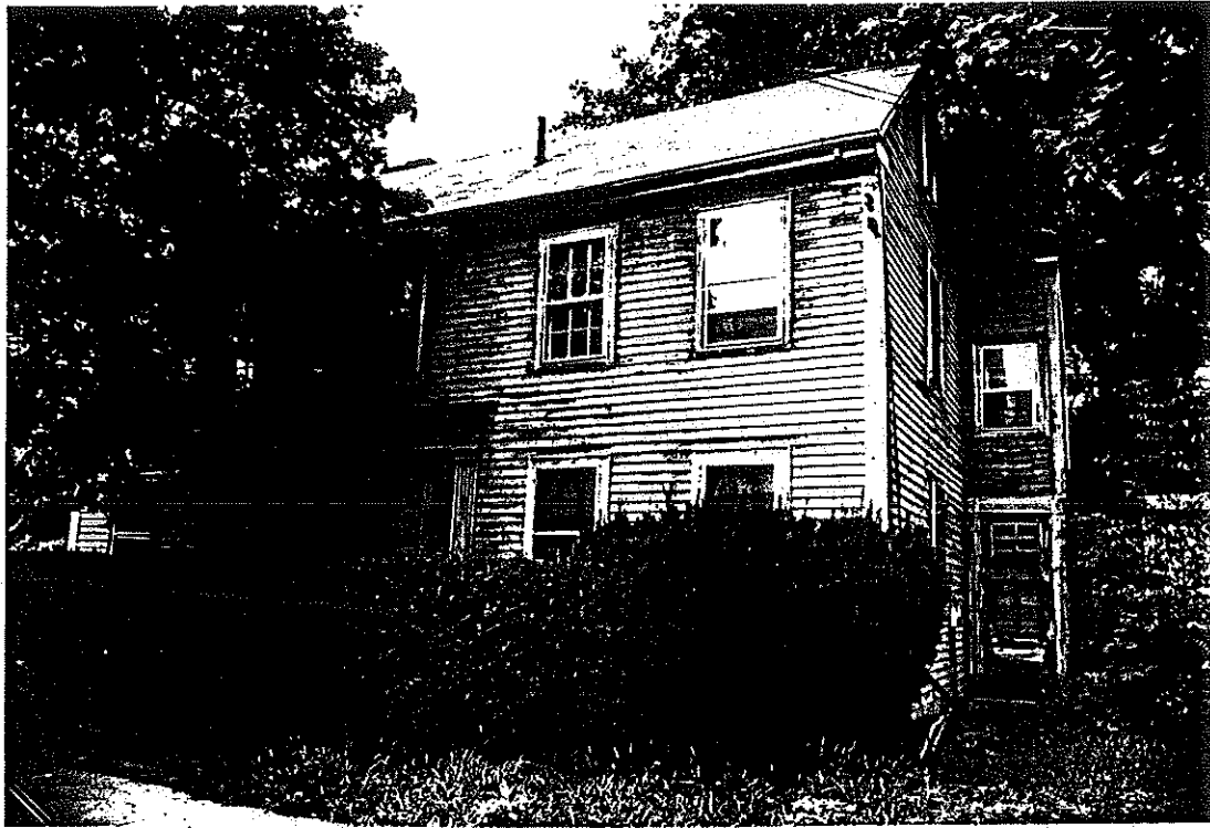
1. The existing front elevation at 1146 Massachusetts Avenue after the aluminum siding had been removed.
