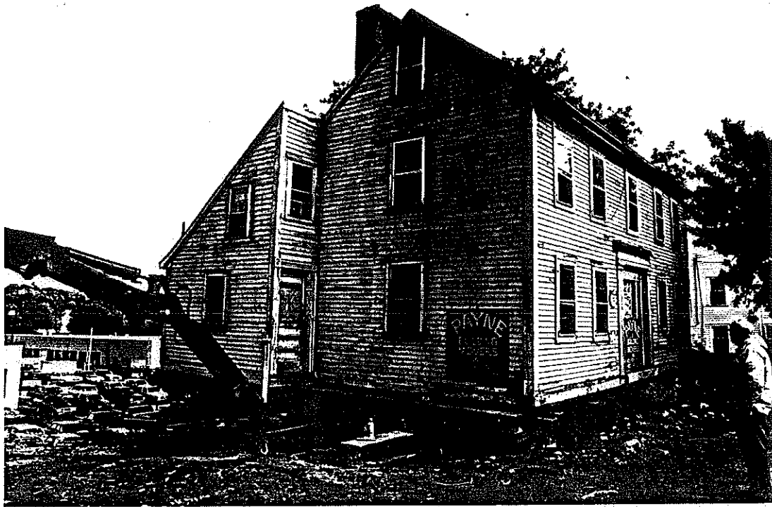
5. Gribbing steel in place, dollies about to be installed.
