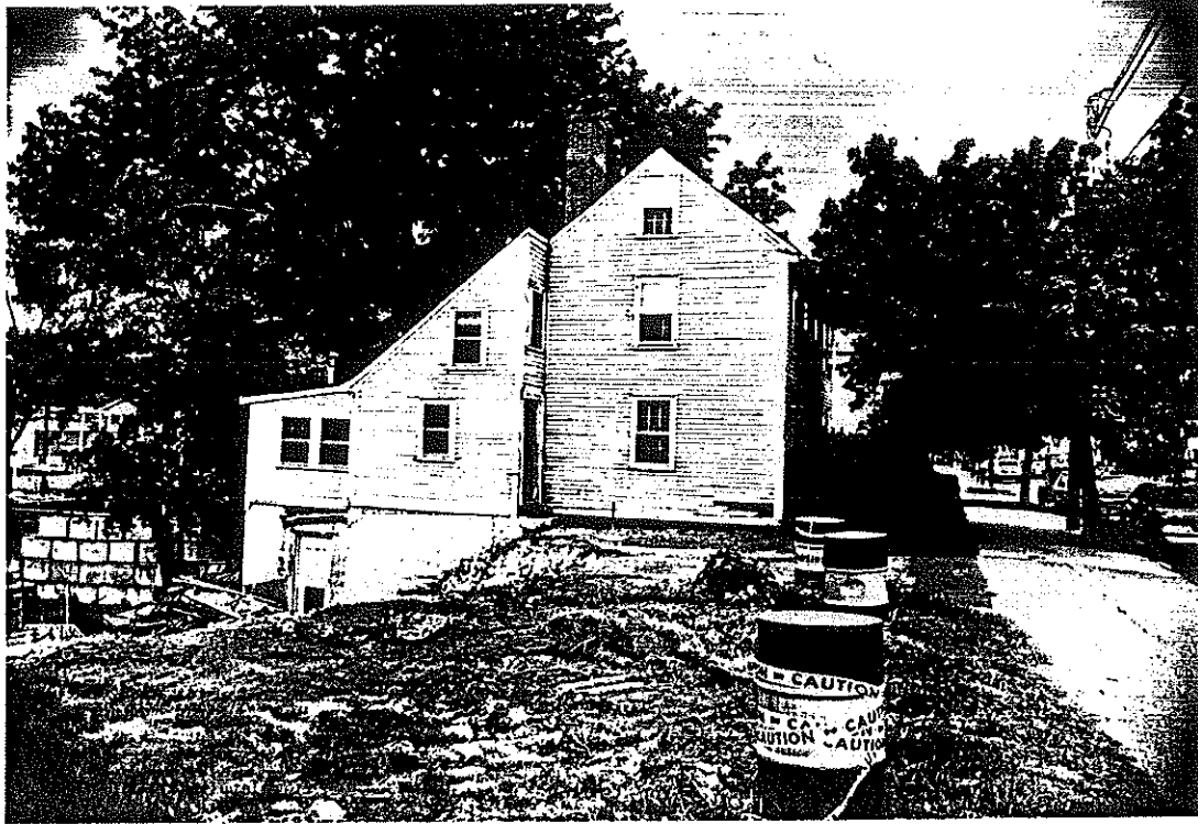
3. West elevation at previous site showing rear addition to be removed.
