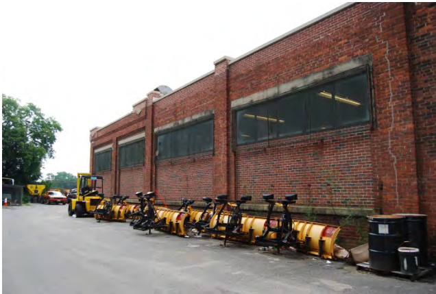
Snow plows stored outside along Building D.
