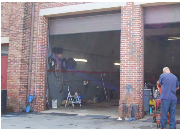
Damaged brick at the maintenance bays of Building D. Concrete window headers show wear; signs of water damage evident.
