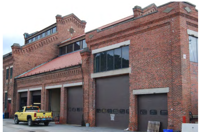
Good tile condition on the North side of the building.
