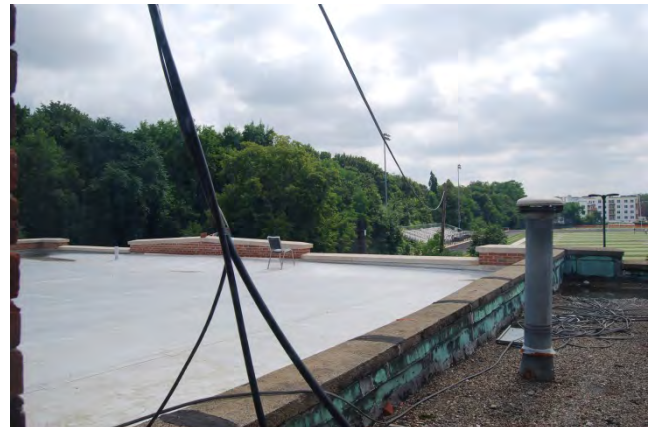
Recently replaced roofing and coping.
