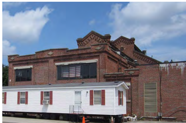
Damaged brick at the maintenance bays of Building D. Concrete window headers show wear; signs of water damage evident.
