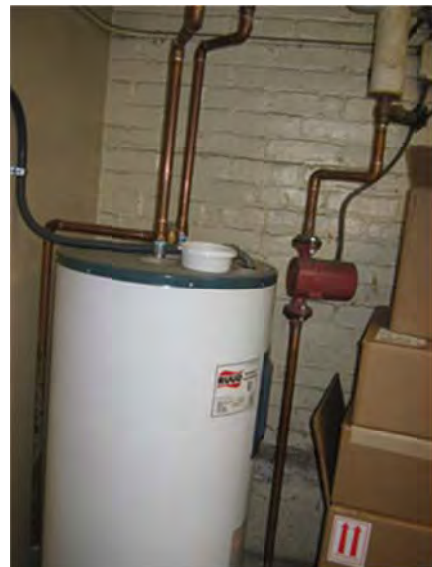
Numerous electric water heaters provide water to hand sinks and fixtures throughout the site.
