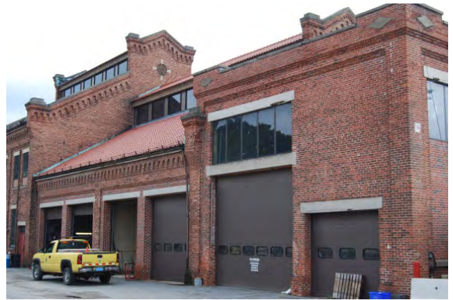
1914 Power Building (Building D)
