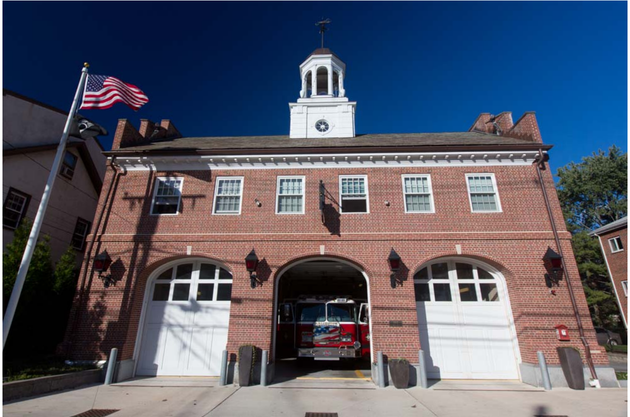
Highland Fire Station
