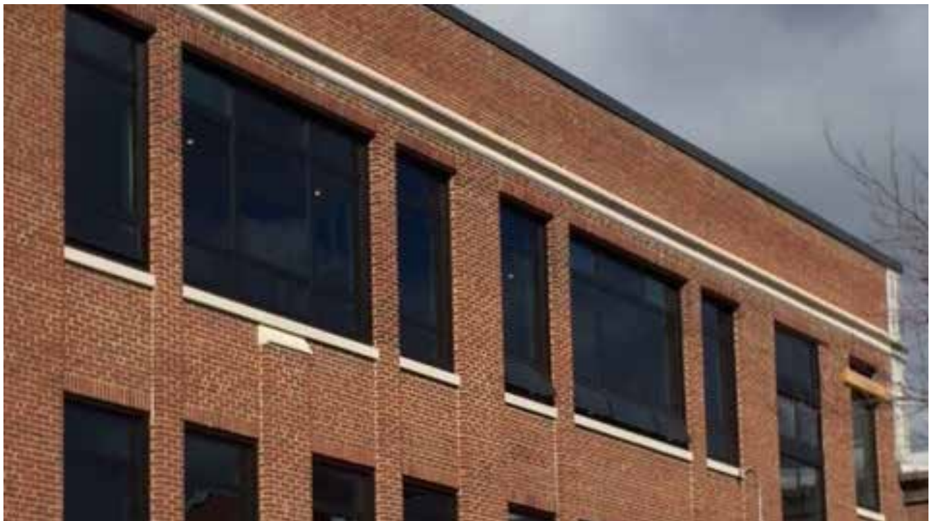
New windows at Gibbs School
