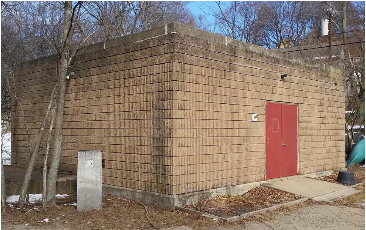
Reservoir pumphouse for bathing beach, slated for gut renovation
